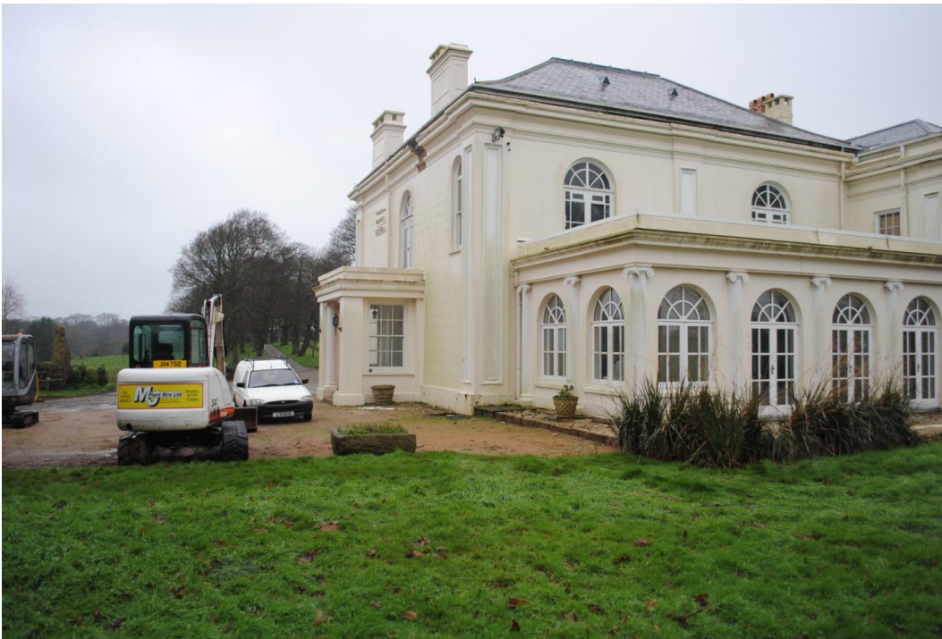
Photo 1: Current property of Diélament , showing 1980s extension (fore) and area of proposed basement and western extension. Looking north.
