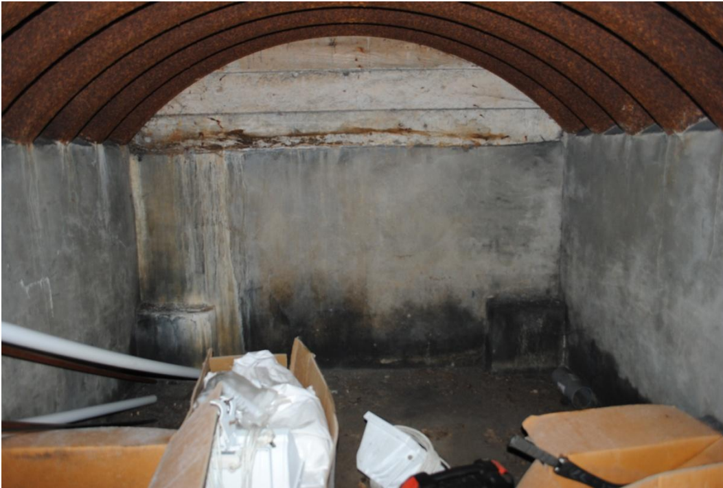
Photo 5: Internal view of subterranean bunker
