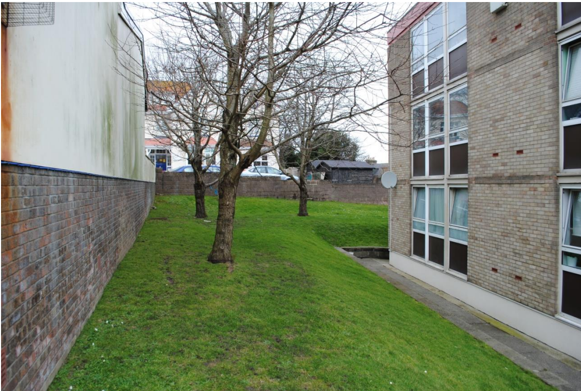
Photo 5: View looking north towards raised grass area. Photo shows terracing to the east (right) to facilitate low rise flats.
