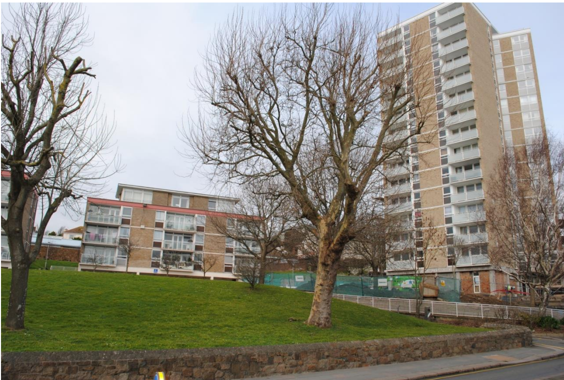
Photo 8: View looking NW showing groundworks associated with high rise and raised grassed area in the background
