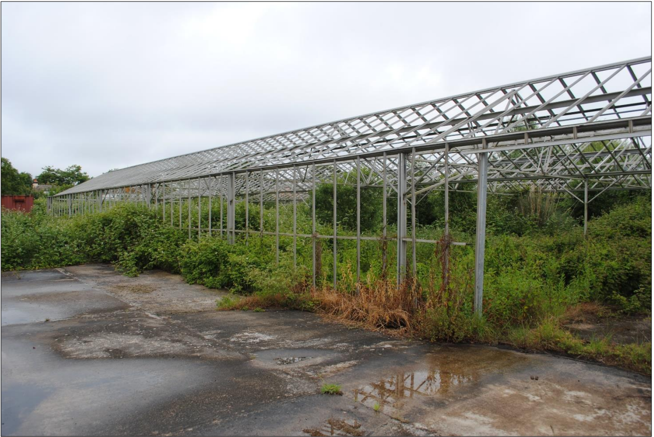
Photograph 4 NE facing view of north greenhouse
