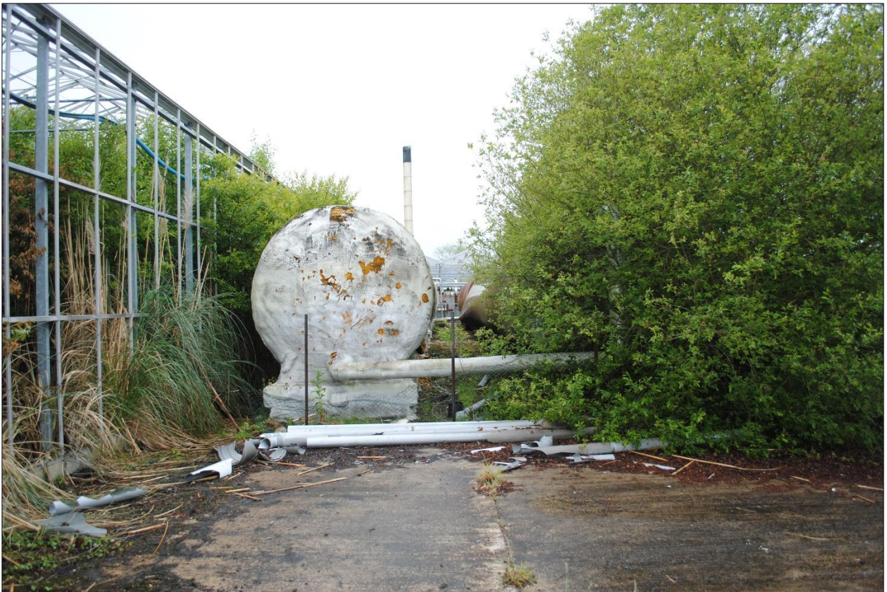
Photograph 3 West facing view of fuel tank
