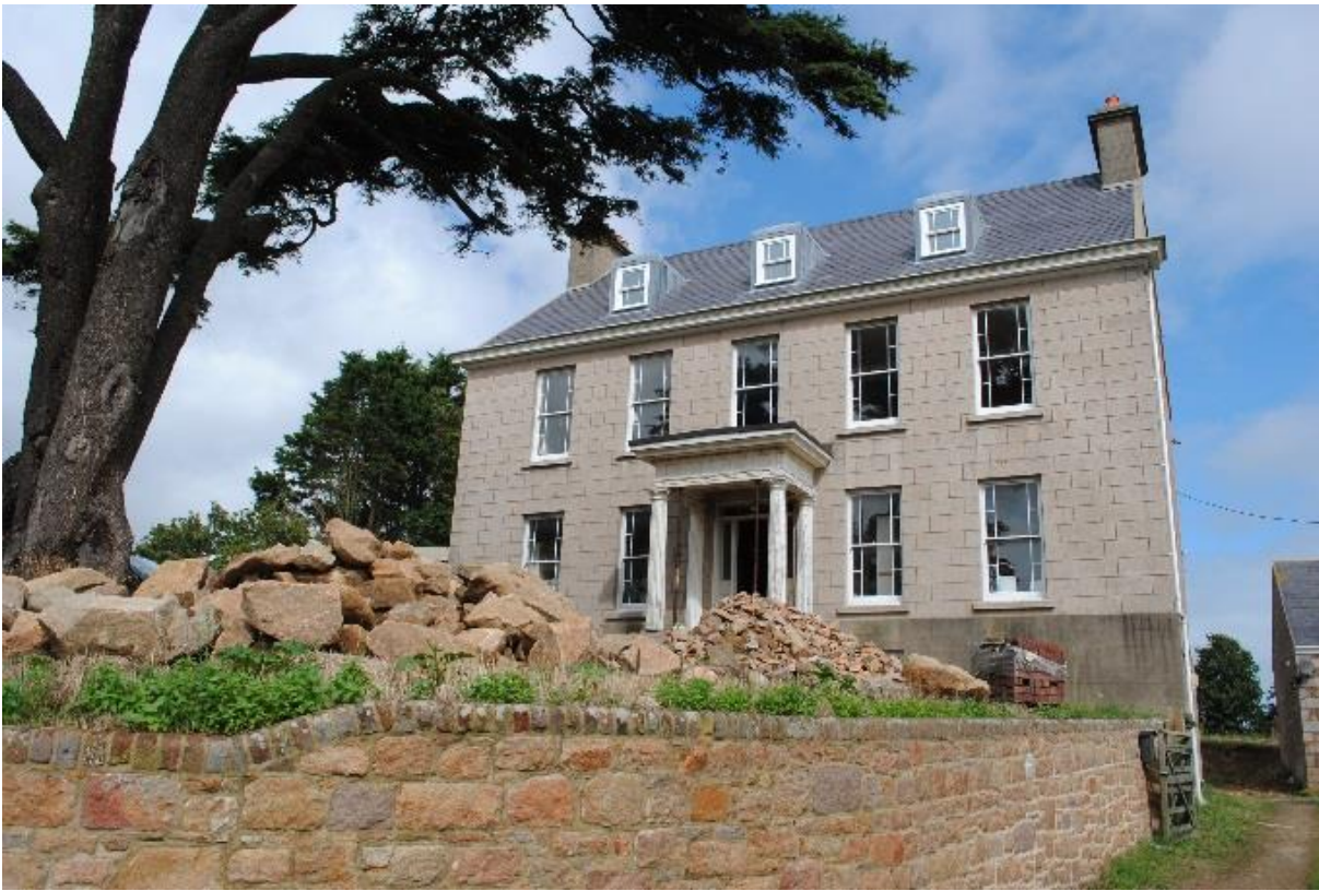
Photo 1: Front of Manor House built in 1873
