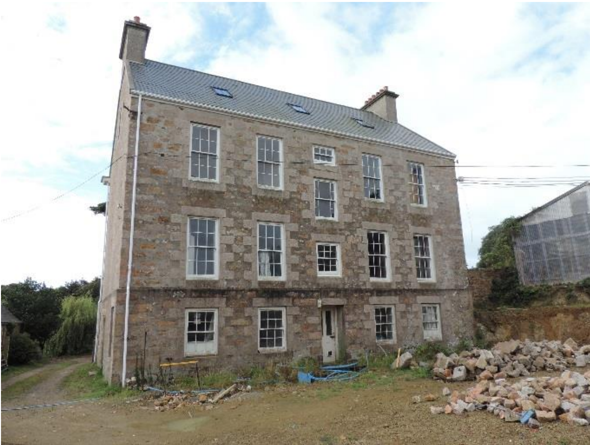
Photo 2: Rear of Manor House (north facing), showing exposed bedrock to the right into which the house was cut
