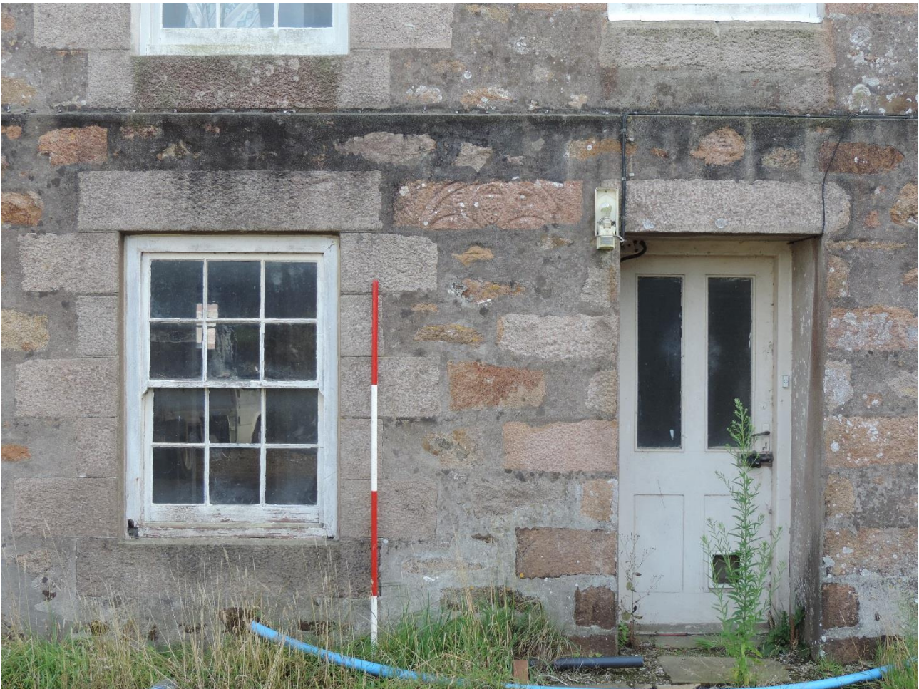
Photo 7: Carved lintel reused in the north wall of the property rebuilt in 1873
