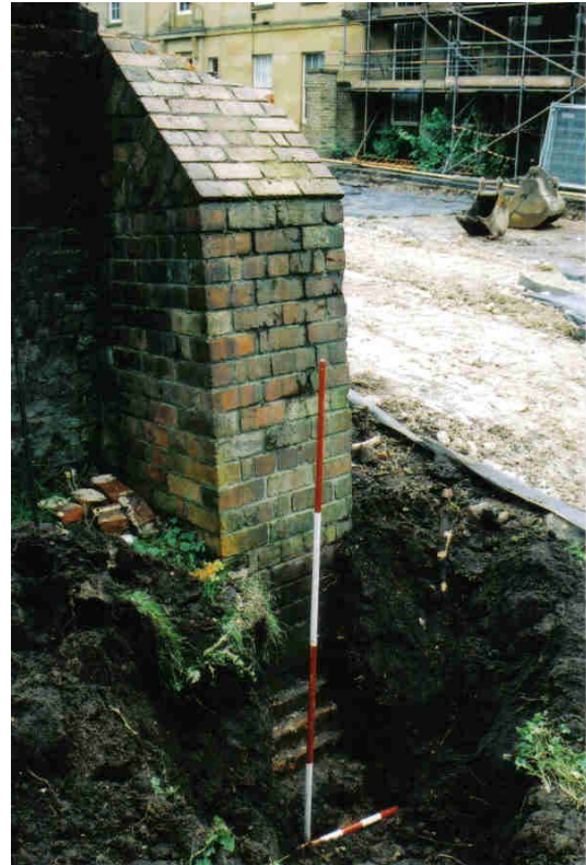
PHOTOGRAPH 4 DETAIL OF BUTRESS F1022 SCALES 2m 7 500mm
