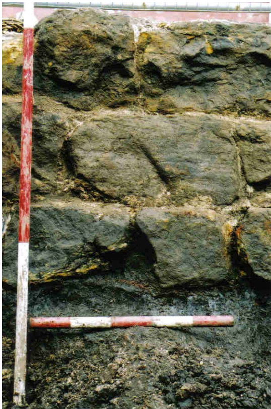
PHOTOGRAPH 3 DETAIL OF BLOCKS IN WALL F1004 SCALES 1m & 500mm
