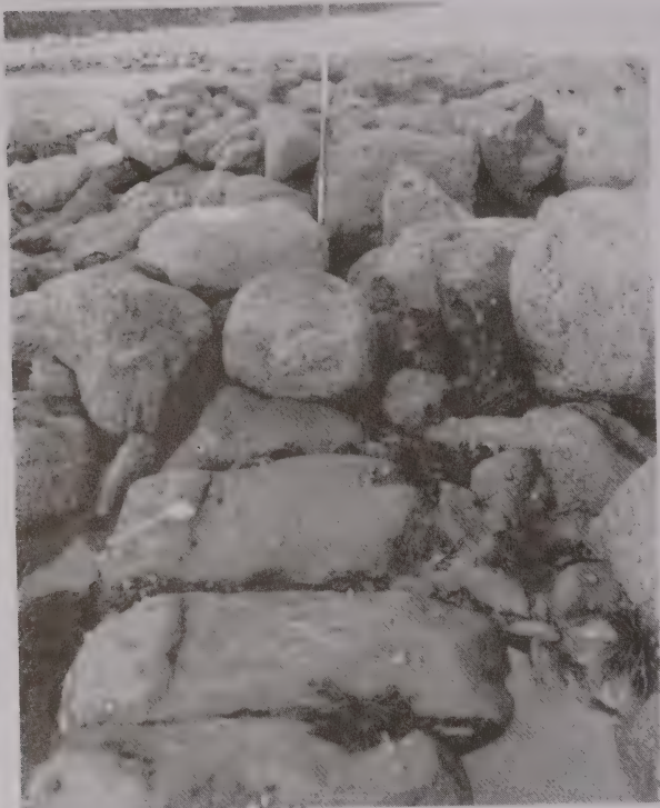
PLATE 7 Looking along part of the inner edge of the north section of the alum house breakwater. Note the retaining 'lips' cut into the top of the blocks. Scale 2 metres length
