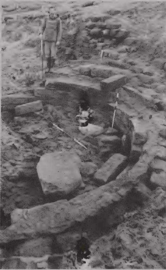
PLATE 6 Part of the perimeter of the circular cistern of the alum house during excavation. Note the clay lining between the inner and outer skins. Scales 2 and 1 metre
