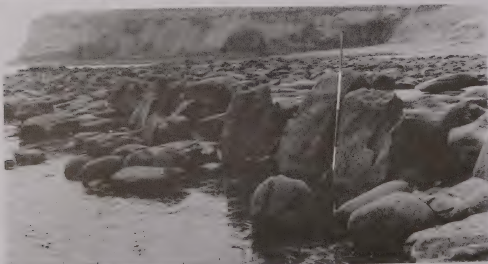
PLATE 8 The outer vertical wall protecting the north section of the alum house breakwater (023). (Scale 2 metres length)
