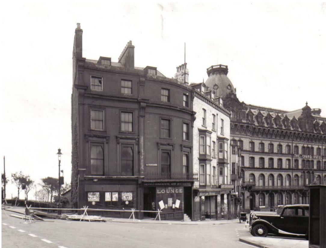
The site on 9 October 1939 as demolition of The Lounge commences
