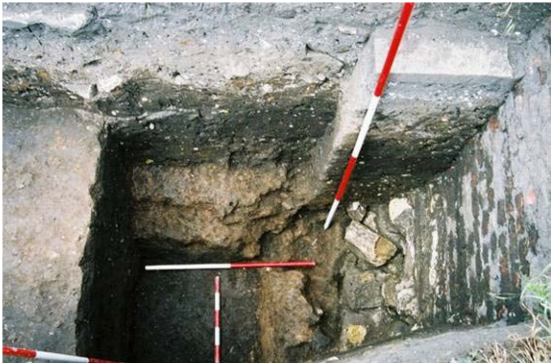
5.Trench 1 looking north showing the footings of the boundary wall Scales 2 metres, 1 metre and 500mm
