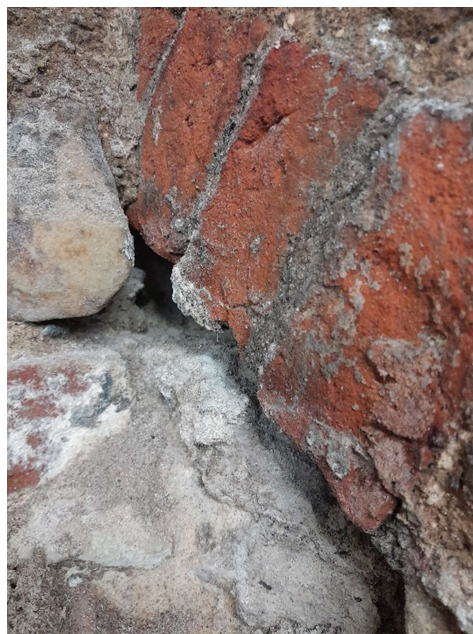
Detail of the fragment of arch at the junction between the north and west walls
