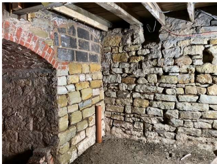
The east wall showing the junction with the north wall and the difference in the masonry between the two walls
