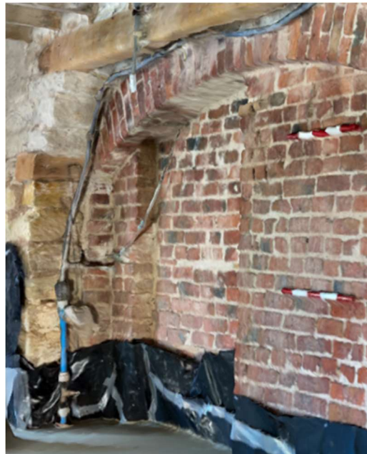
Oblique view of the corbelling 'C'
