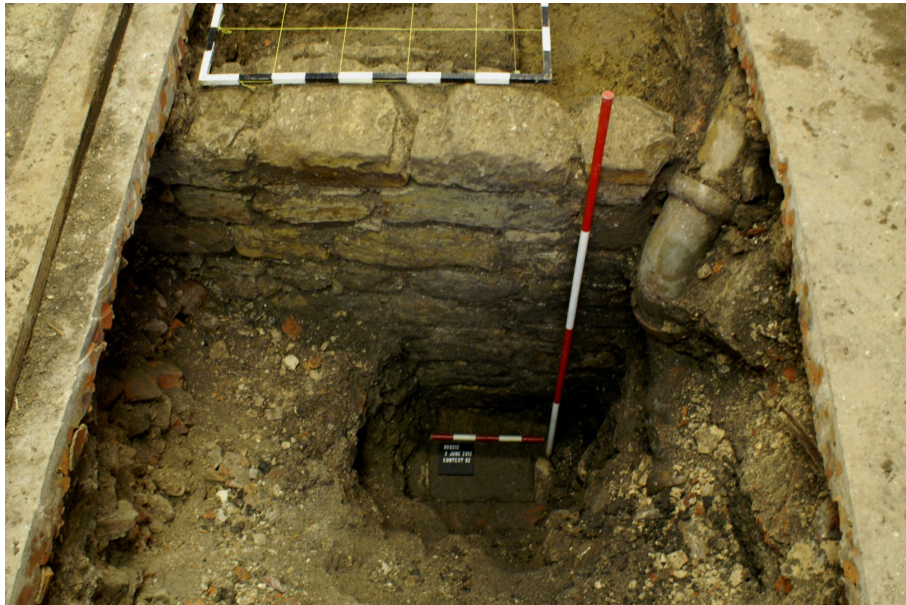
Plate 4. Trench 2 looking north showing wall F55, drain F68, sondage into cellar fill and the cellar floor
