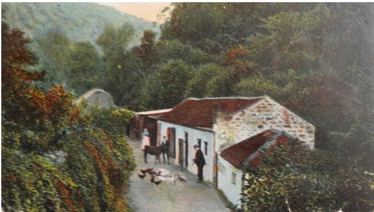
Figure 10. Building 2 viewed from the north-east in the early 20th century.
