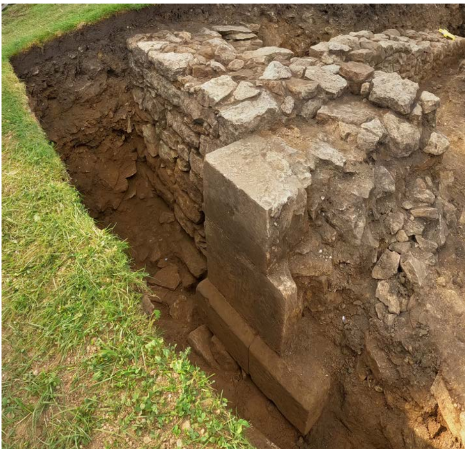
Figure 12. View looking west of south wall of Building 2 showing the ashlar plinth. (Photograph S. Gandolfi)
