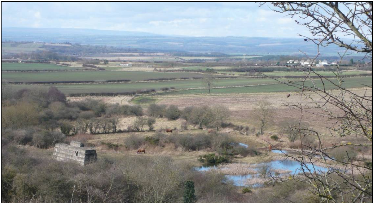
Plate 5: View out over the Phase III colliery site showing the remains of the head gear known now as 'the castle' with the former Crowtrees Railway just to the right, marked by a line of the trees.
