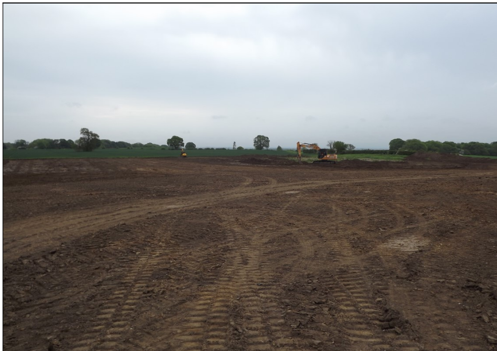
Plate 1. General view of site, looking south-east
