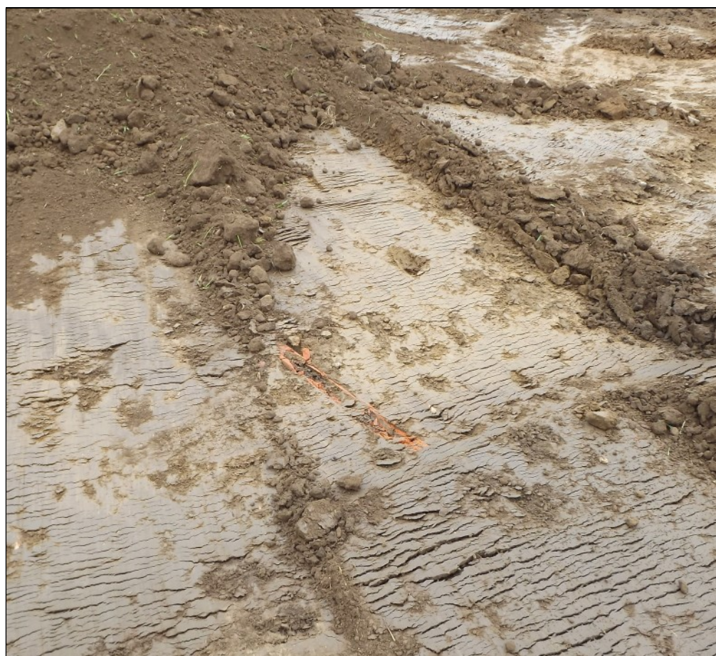
Plate 2. Example of the remains of land drains
