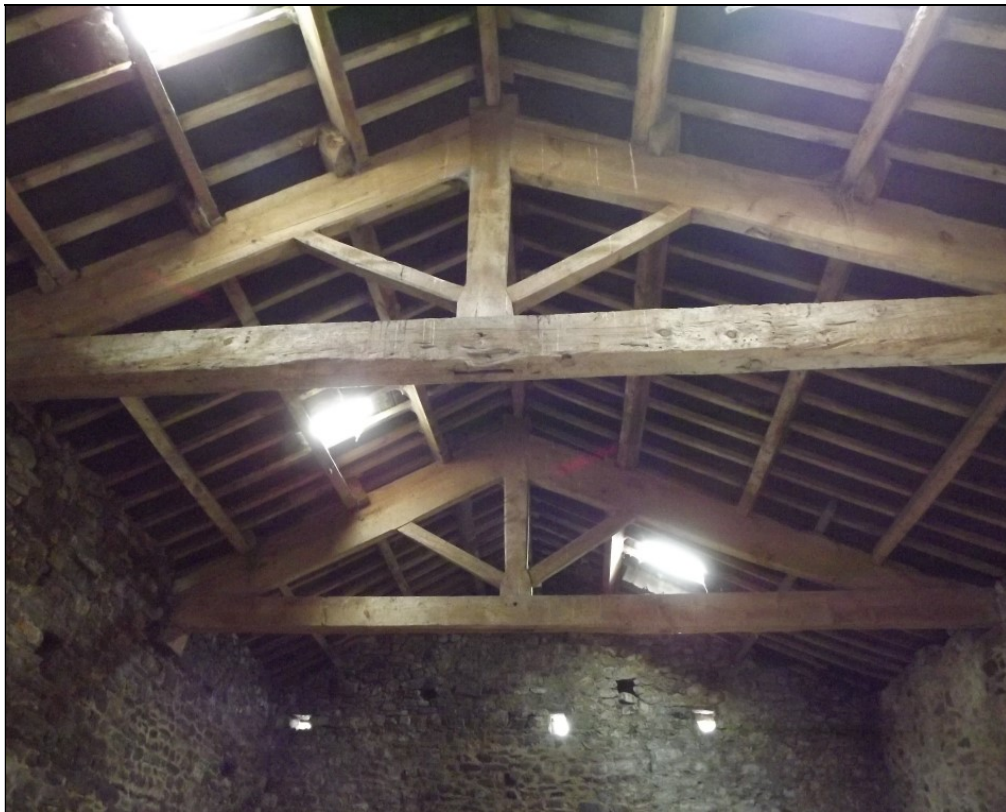
Plate 11. Later, pegged trusses at the eastern end of the barn, looking east
