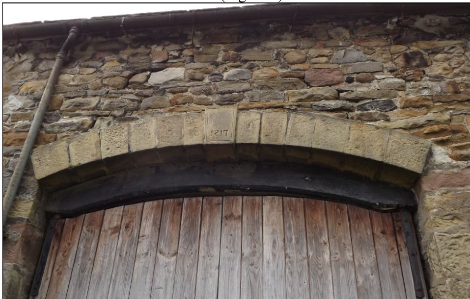
Plate 8. Dated key stone and rebuilt arch, looking south
