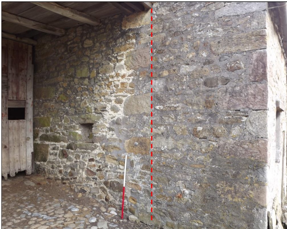
Plate 6. Lantern niche & butt join of Phase II extension, looking NE, scale 1m
