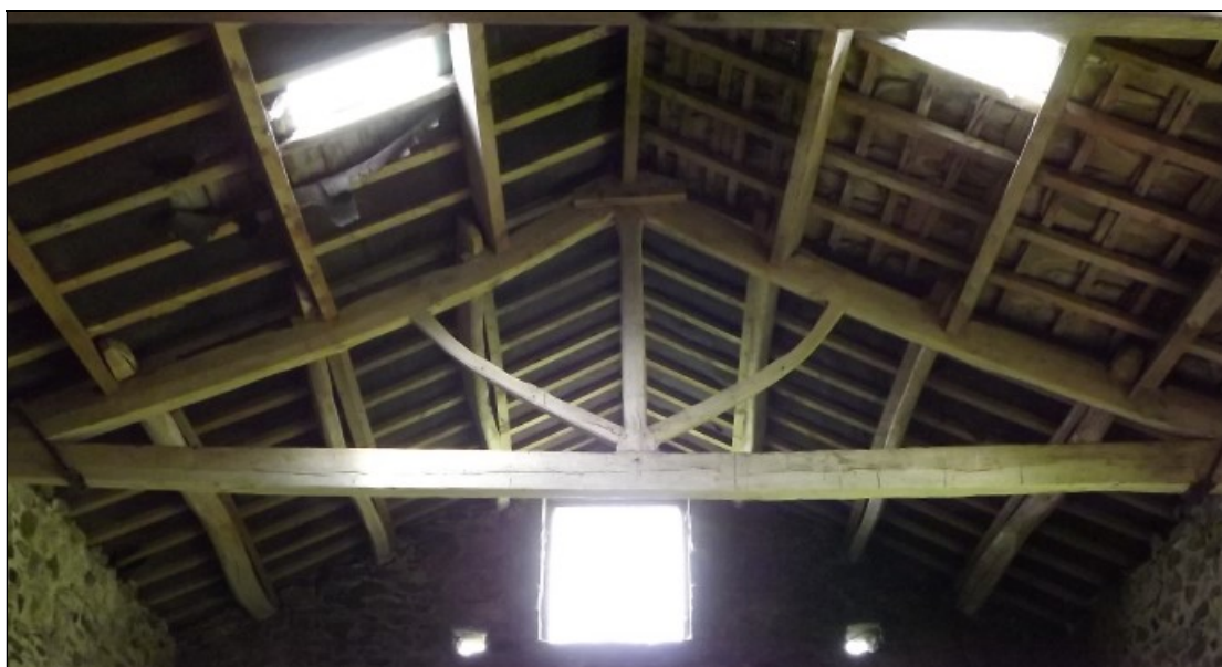
Plate 3. King post truss with curved braces at west end of the barn, looking W
