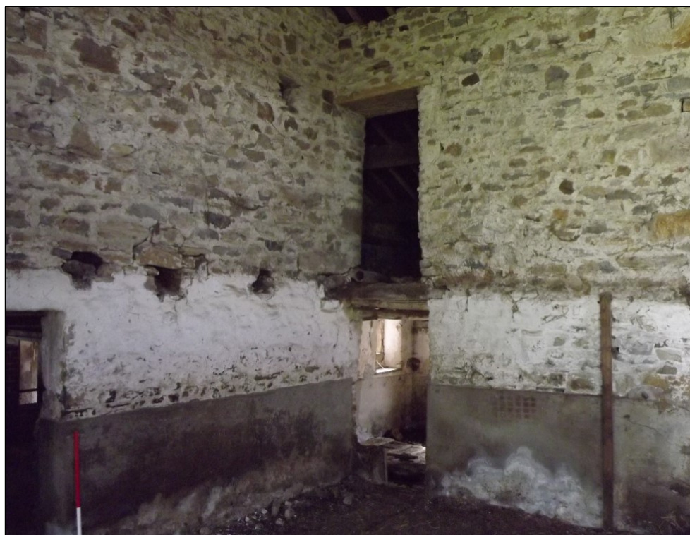
Plate 4. Joist holes and 'tide mark' showing hayloft, looking SE, scale 1m
