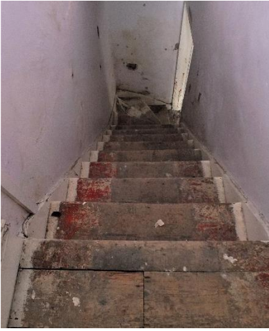
Stairs from upper landing
