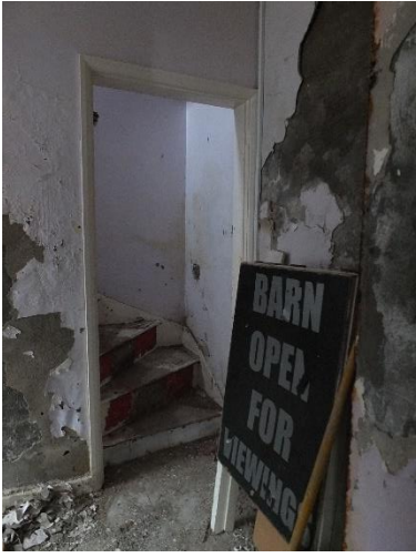
Room looking towards stairs
