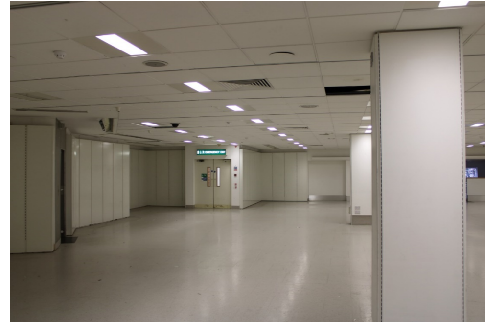
Photo 22: View east across northern side of floor towards northern staircase to rear, window on Lister Gate frontage to right and lift visible to left
