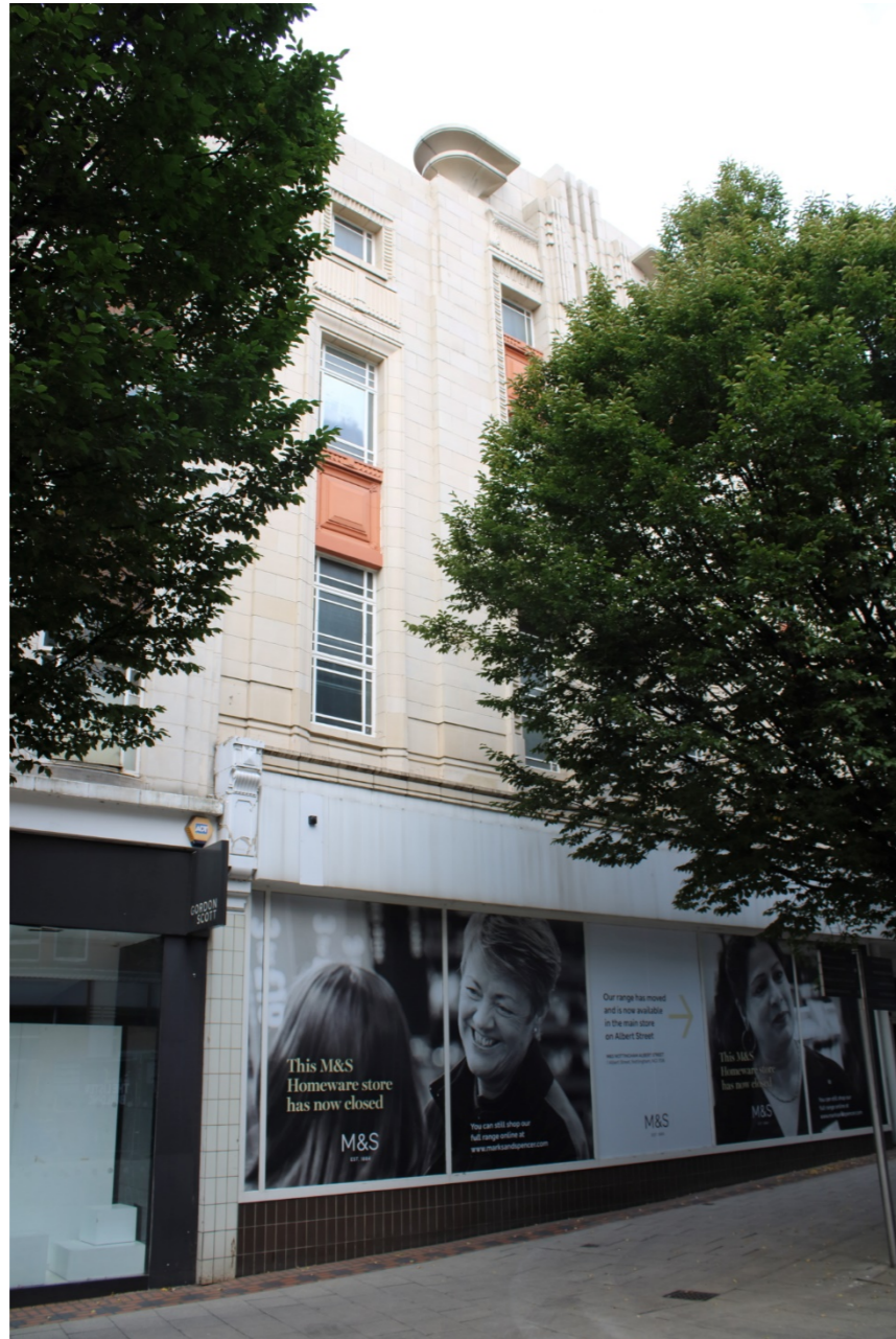
Photo 1: Southern end and side bay above shop front at ground floor
