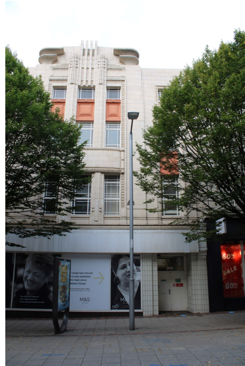
Photo 2: Northern end and side bay above ground floor shop front .
