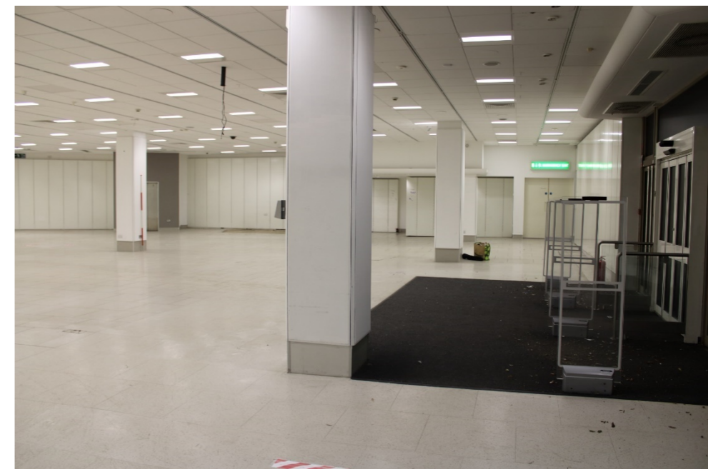
Photo 20: View north across ground floor retail area across entrance to Lister Gate to right with stairwell behind and lift to right
