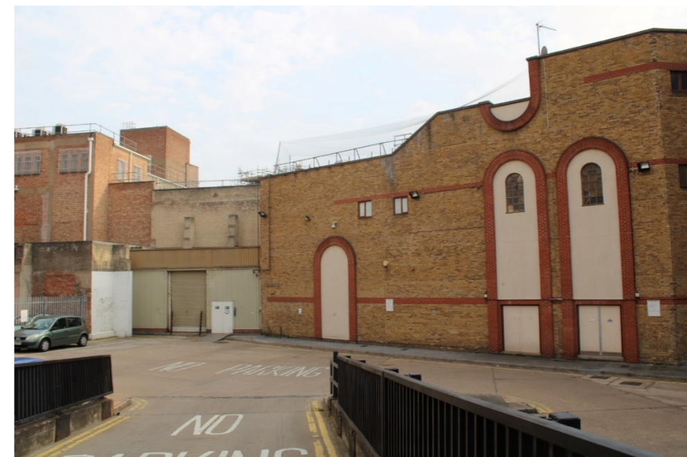
Photo 13: View northeast rear of Nos 22-26 Lister Gate, formed by the modern brick façade with red arched details and store room access to left
