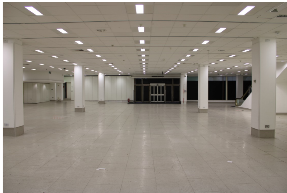
Photo 18: View east across retail area to doorway entrance to Lister Gate, escalator to right and utility room to left (alarm panel/fuses etc)
