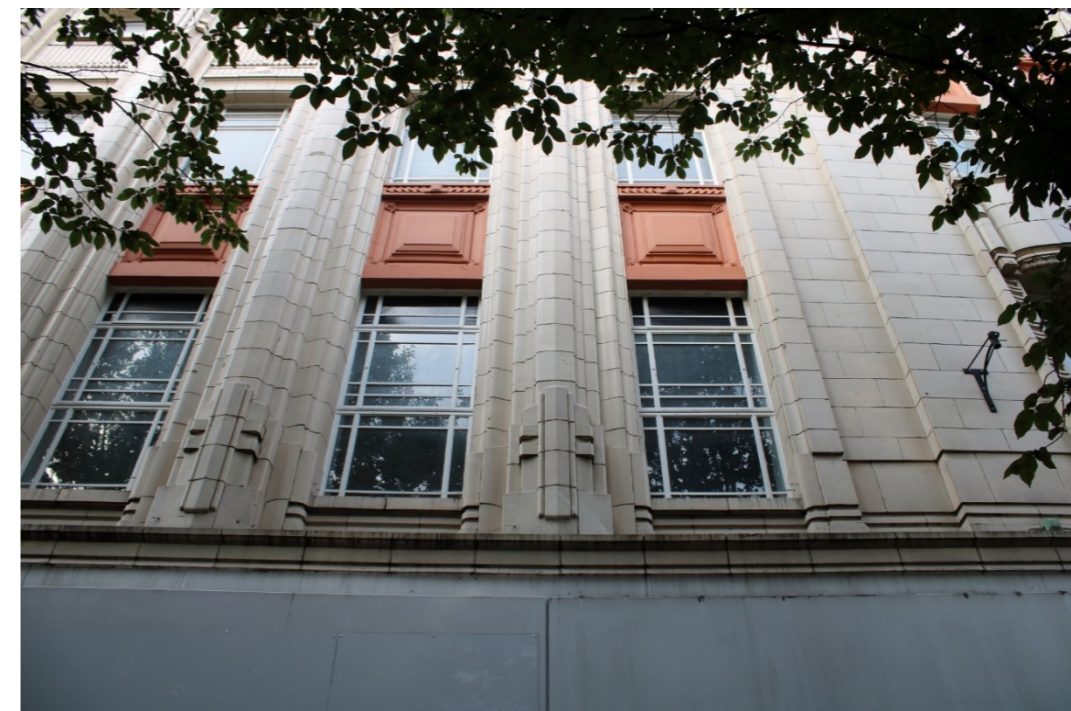
Photo 8: Three windows of central bay (northern window to right)
