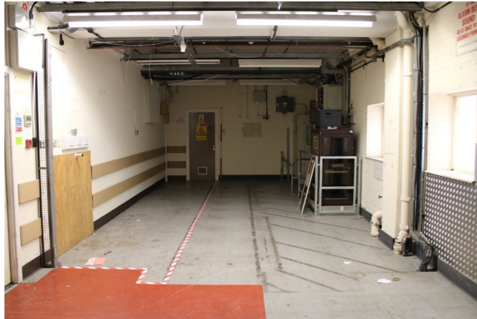
Photo 32: View south along rear storage area to west of first floor retail area plant room to rear, doors to retail area to left and window to yard area to right
