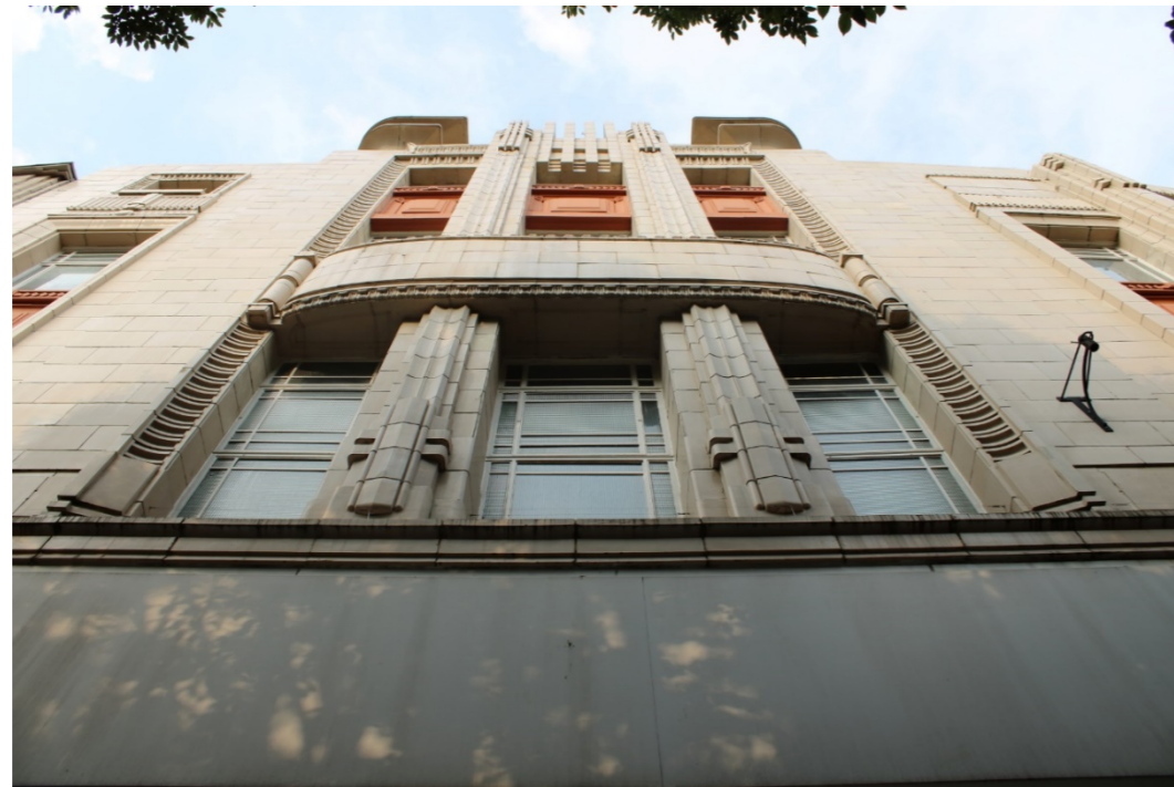
Photo 5: View upwards of the southern side bay, above ground floor
