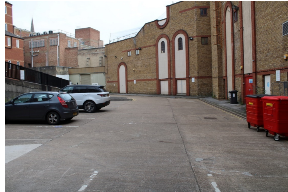
Photo 16: View northeast across proposed extension area to rear of Nos 22-26 Lister Gate
