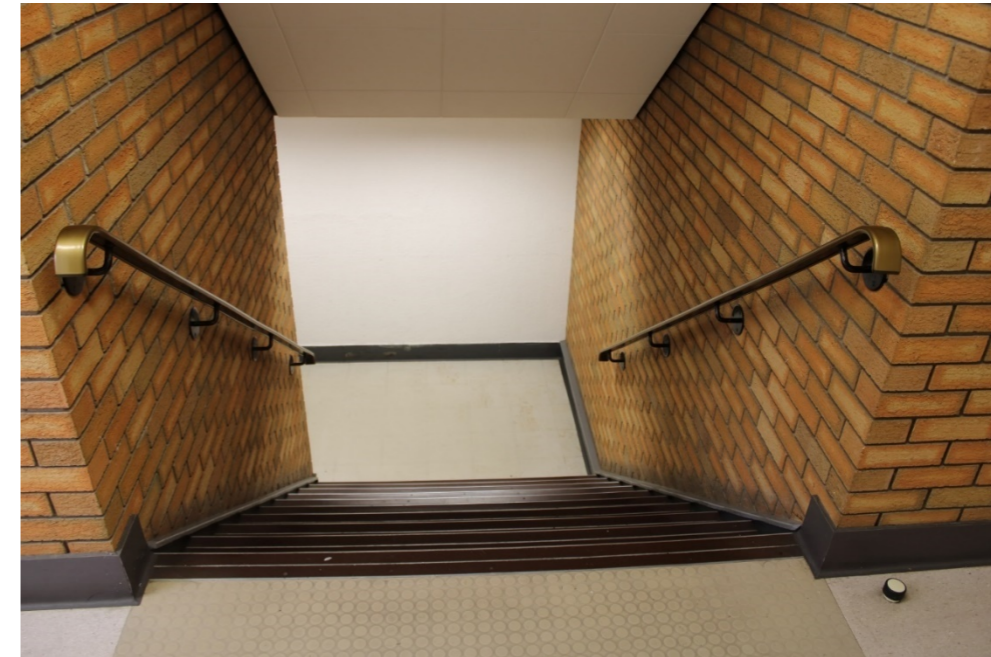
Photo 30: View down western stairwell towards first floor at rear of Building
