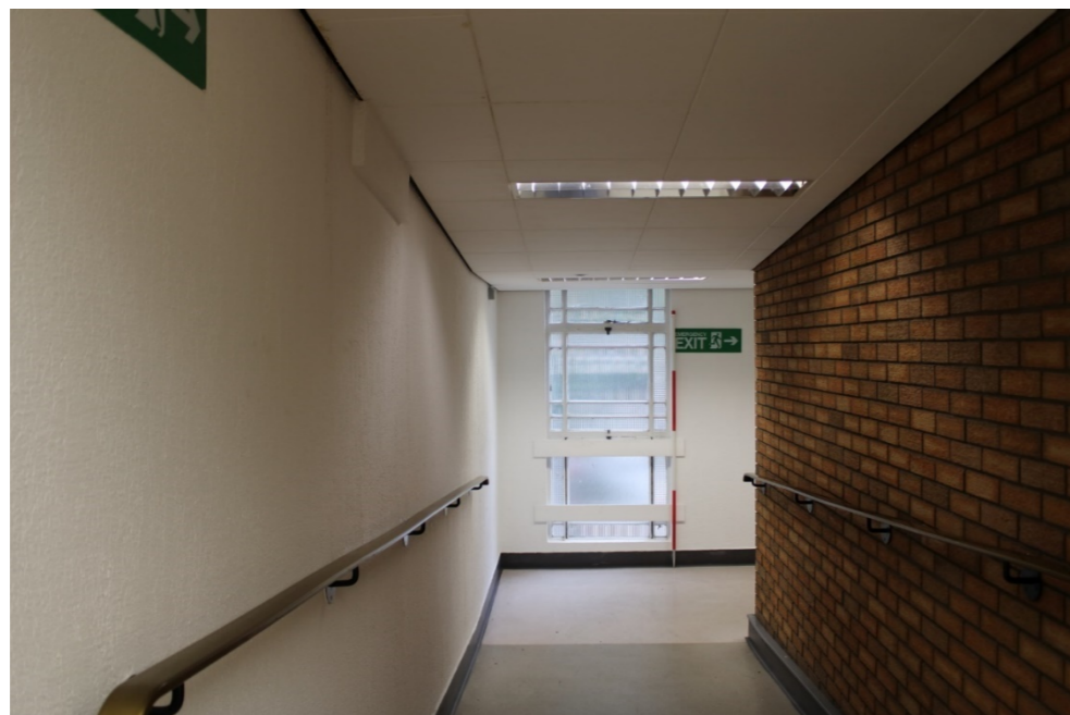
Photo 29: View east of first floor window 13 on northern side bay overlooking Lister Gate, within northern stairwell and showing ramp up to second floor
