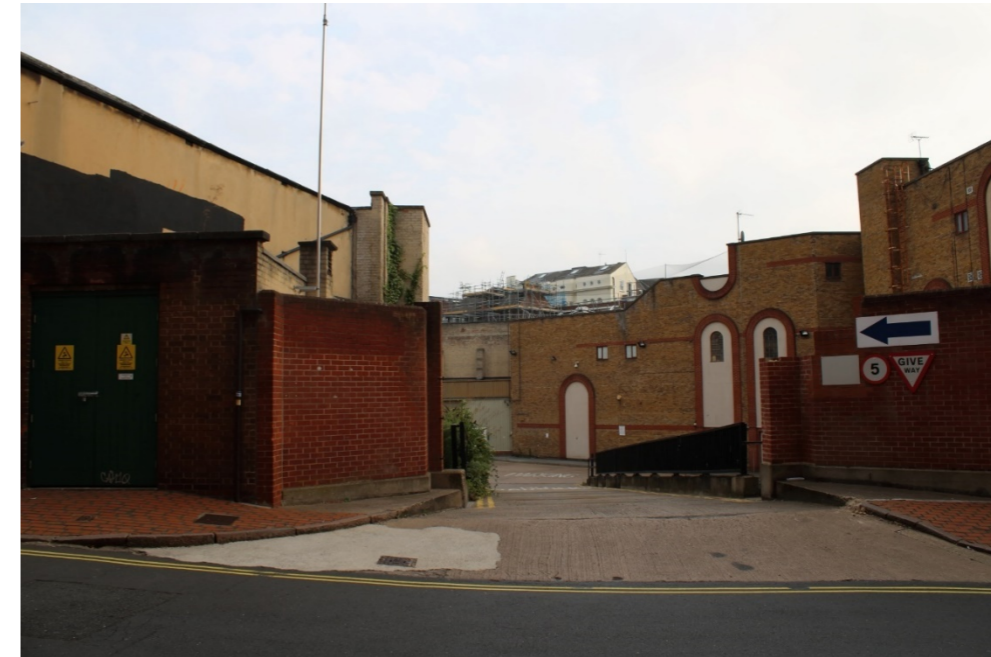
Photo 12: View northeast from Stanford Road showing rear of Nos 22-26 Lister Gate and ramp down from road level.
