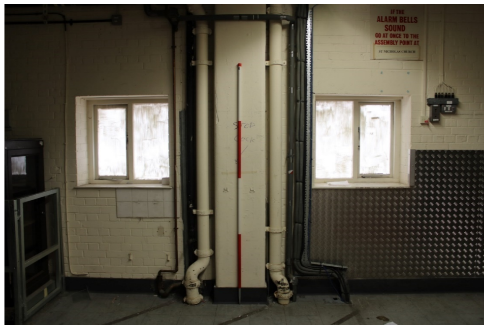
Photo 33: View west of modern windows overlooking rear yard area within storage area to rear of first floor retail space
