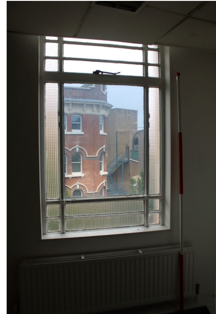
Photo 48: View east of second floor window 1 on Lister Gate frontage within small end office in southeastern corner of building
