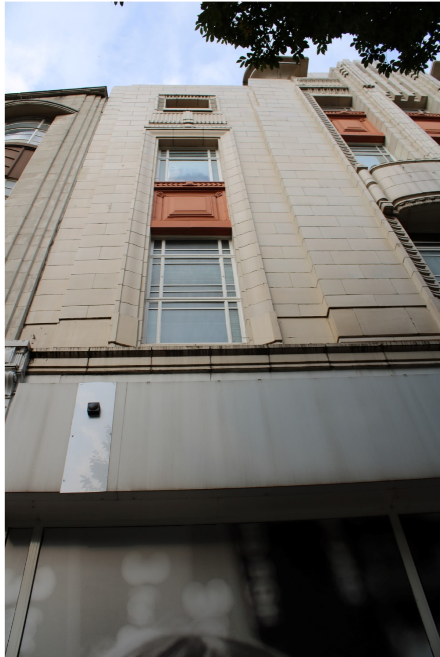
Photo 3: Southern end bay above ground floor shop front
