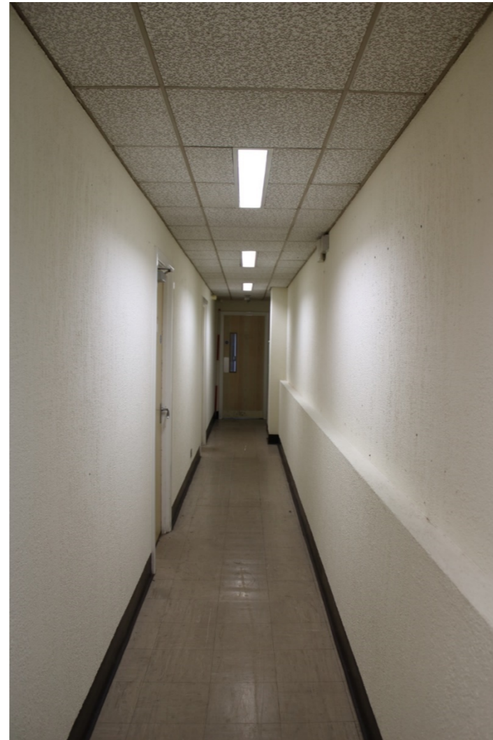
Photo 44: View south along corridor, leading from landing, on western wide of second floor area with doors off leading to offices and staff facilities
