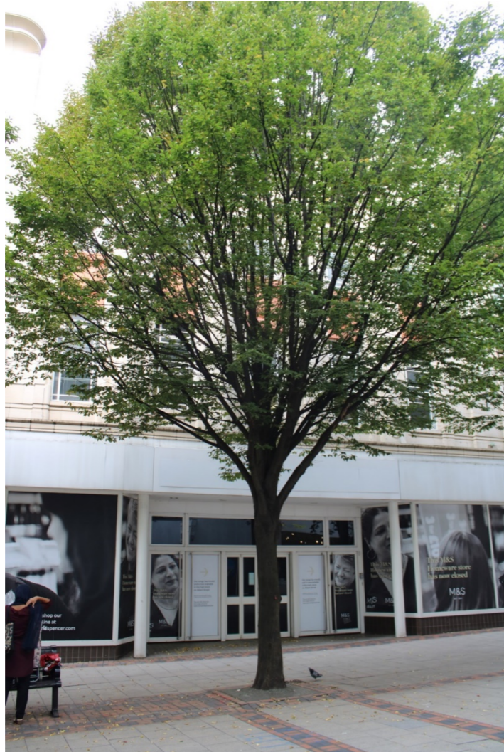
Photo 9: View of main recessed shop front entrance at ground floor
