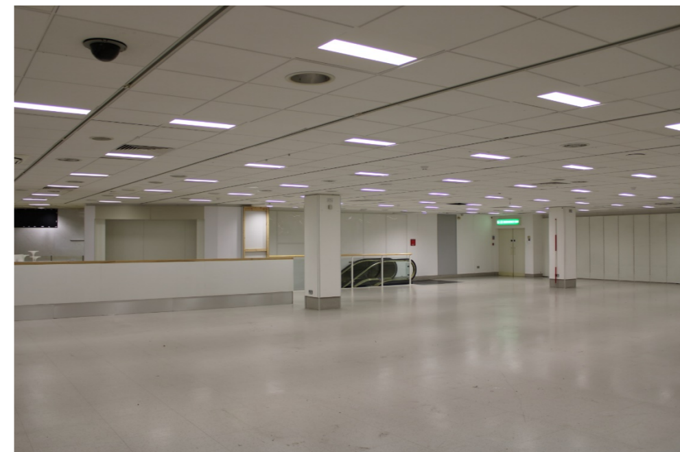
Photo 23: View southeast across first floor showing top of escalator and western stairwell
