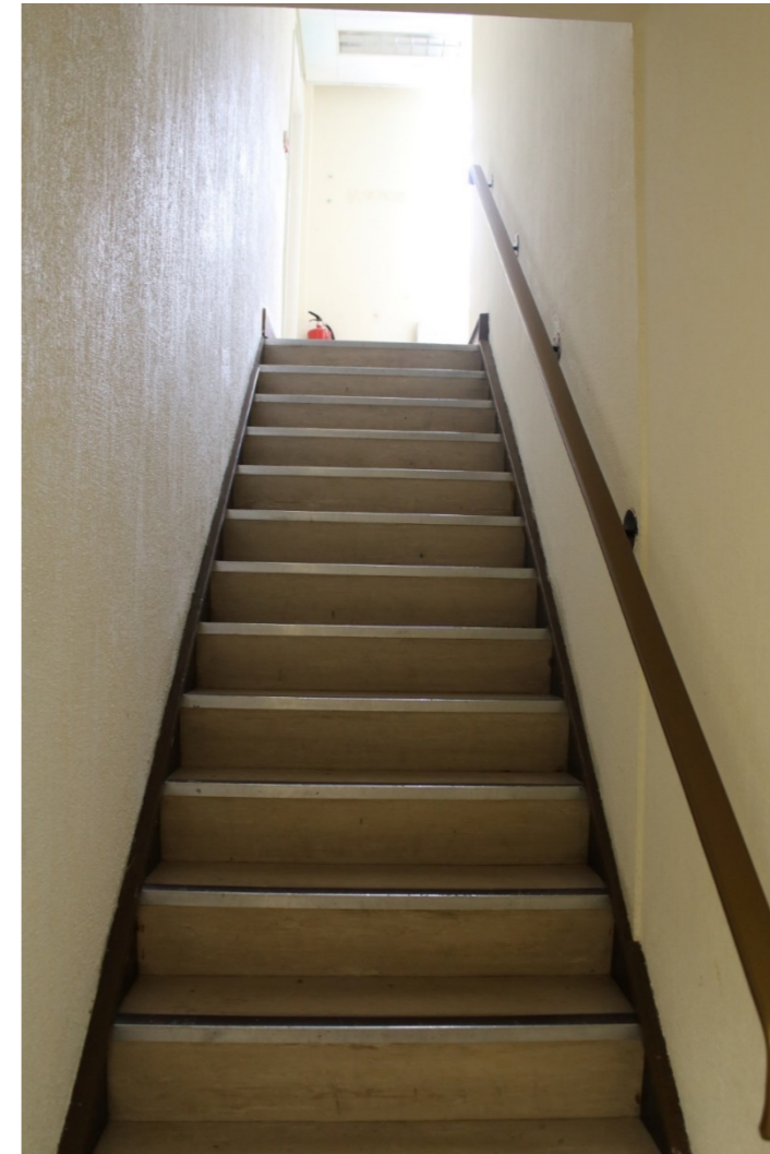
Photo 39: Staircase up to second floor
