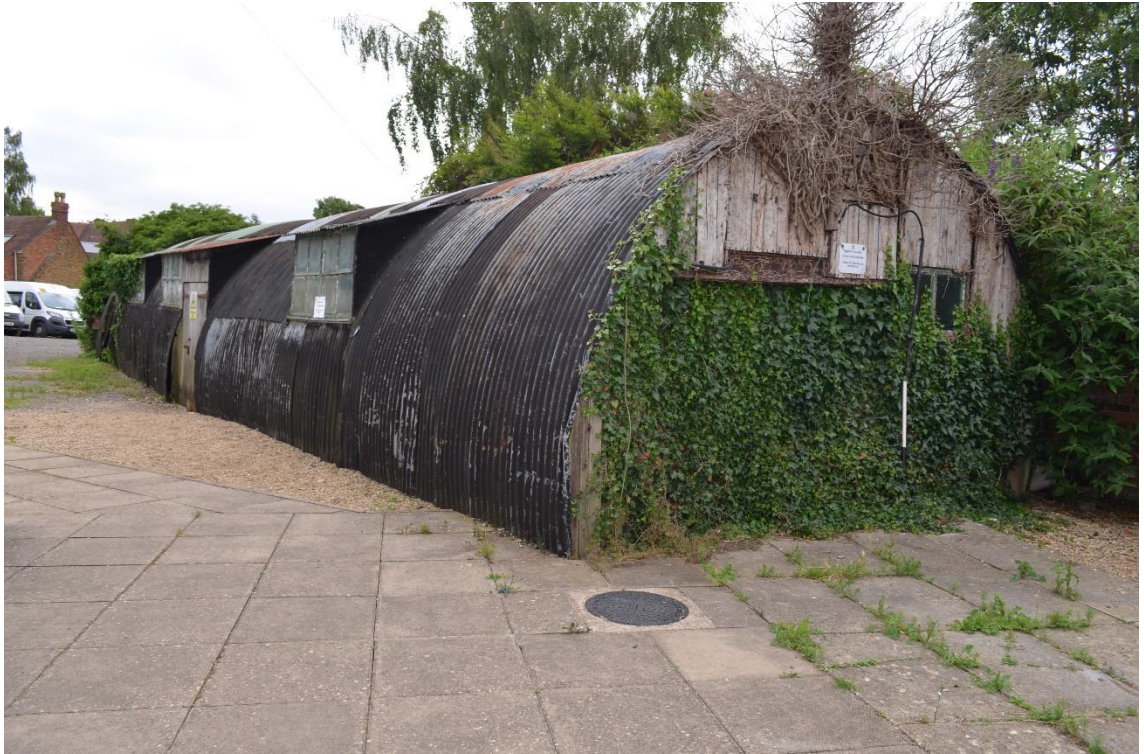
2: Nissen hut from the west looking at the western elevation and showing the projecting dormers. E
