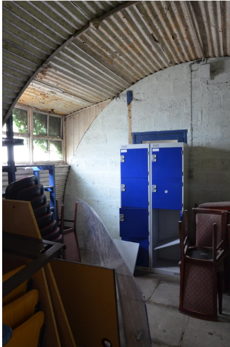
10: Central room, lockers block historic door in concrete block wall. NE
