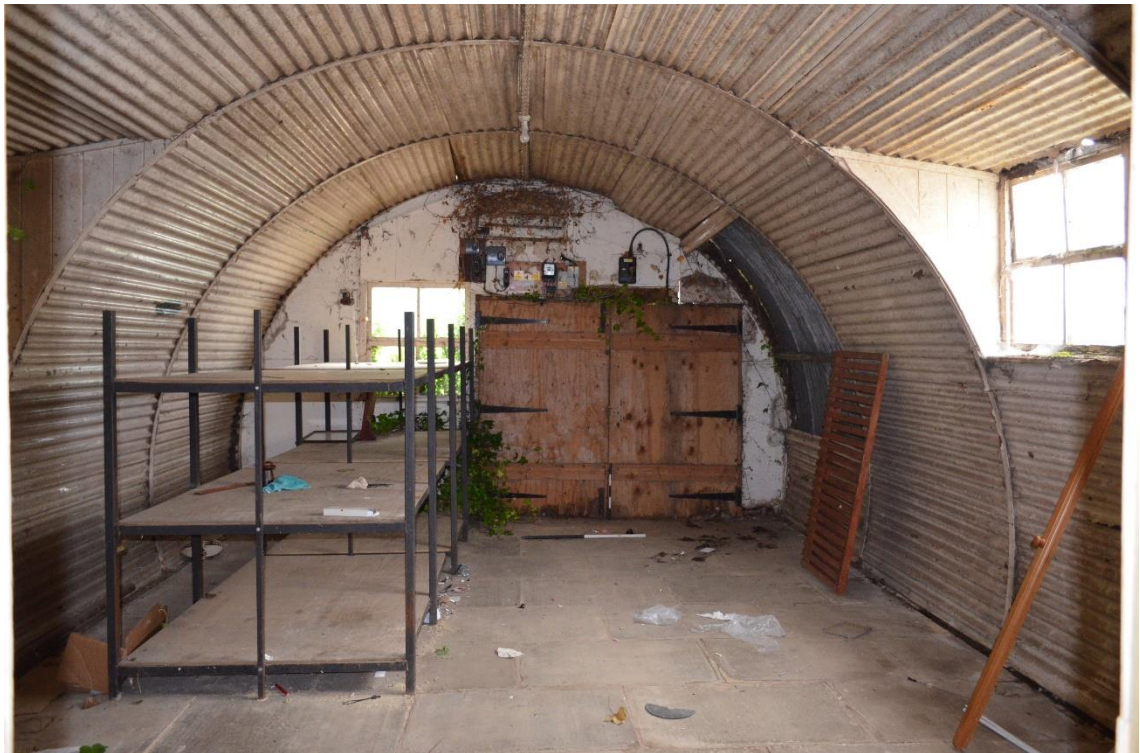
6: Interior of the larger western room. W
