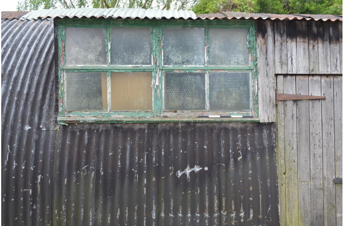
4: Detail of window, standard across the building.
