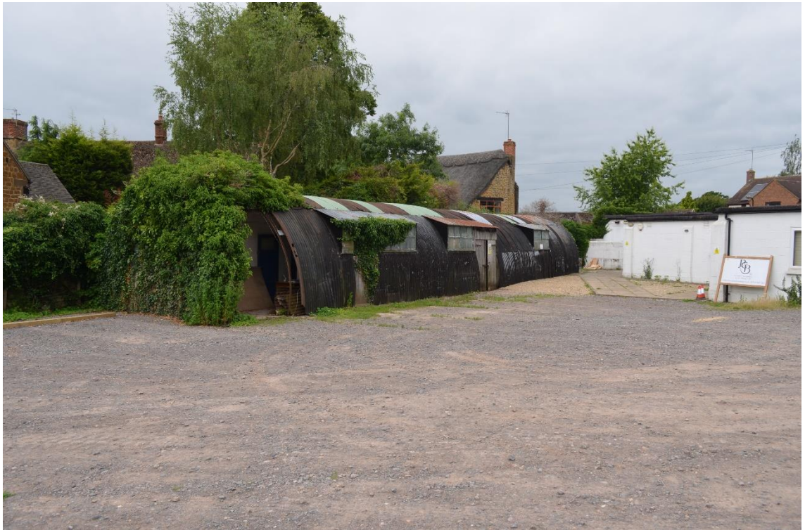
1: The Nissen hut in its context with overgrown eastern elevation. W
