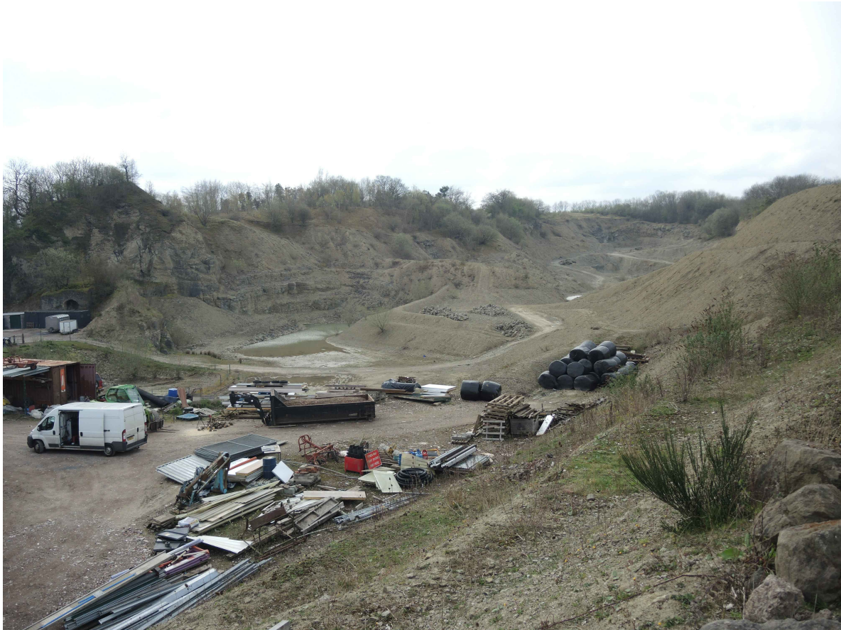
Plate 3: Proposed development area within Farley Quarry from the north (9 April 2019) with lime kilns (S6) to the left
