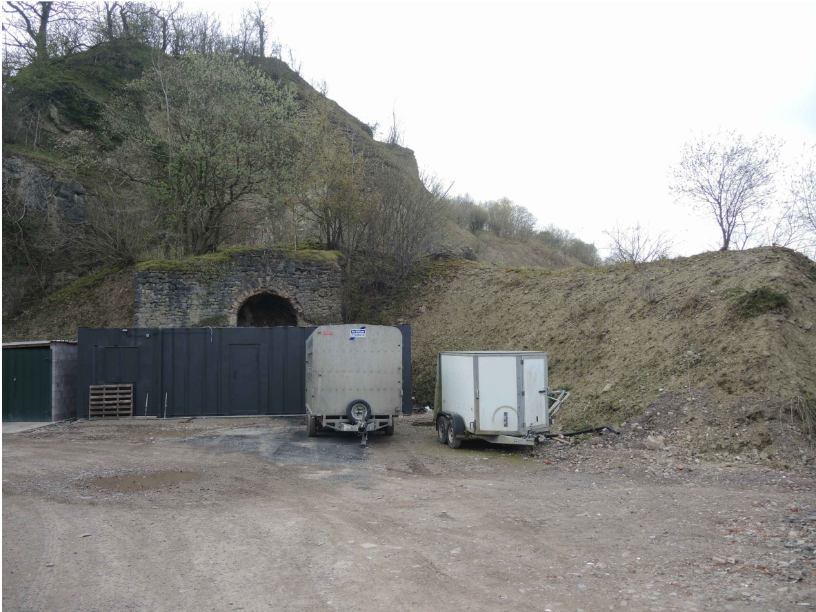
Plate 7: Lime kilns (S6) from the north (9 April 2019)
