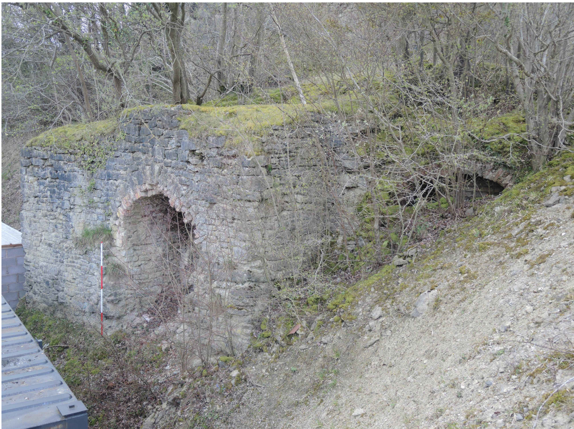
Plate 8: Lime kilns (S6) from the north-west (9 April 2019) 2m scale
