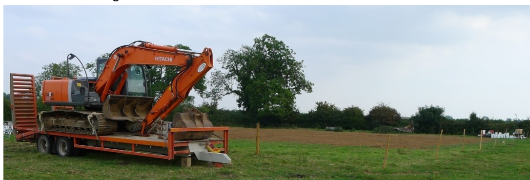
8: Back-filling expertly completed, the 13-ton Hitachi ZX130LCN digger awaits collection
