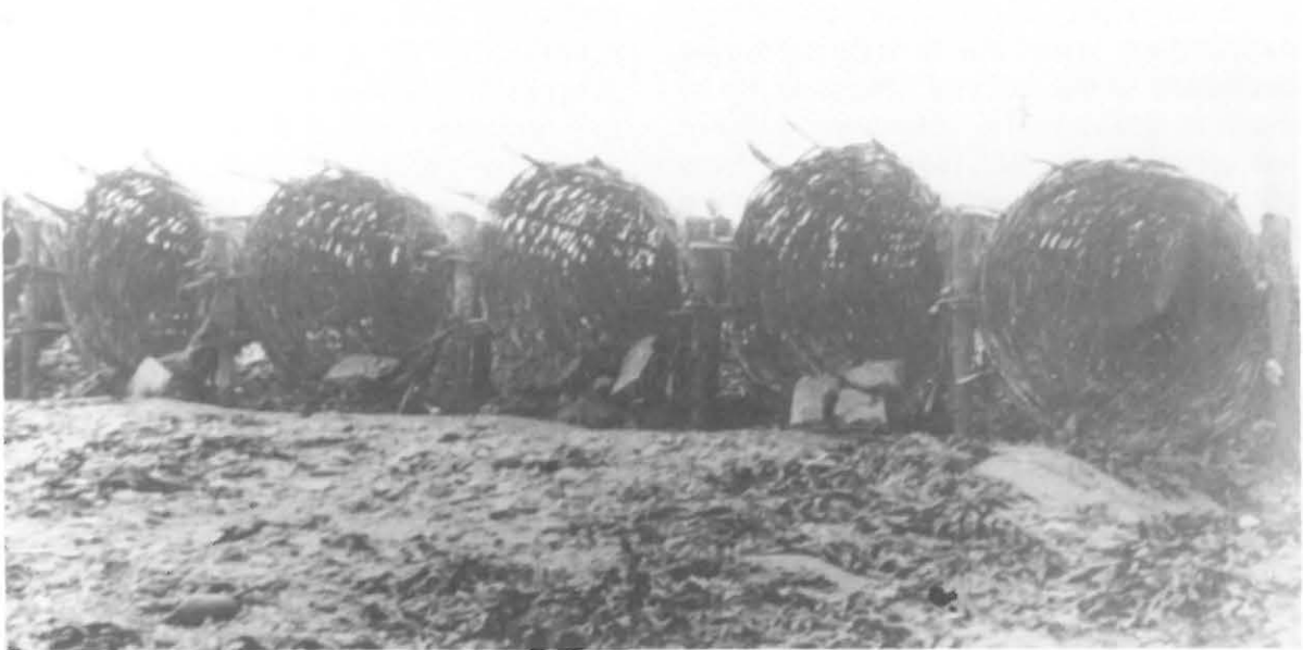
Figure 31. Putt weir at Goldcliff, 12th May 1938 (Note 2). Front view showing putt entrances. Diameter 1.3 m. Facing the ebb tide.
