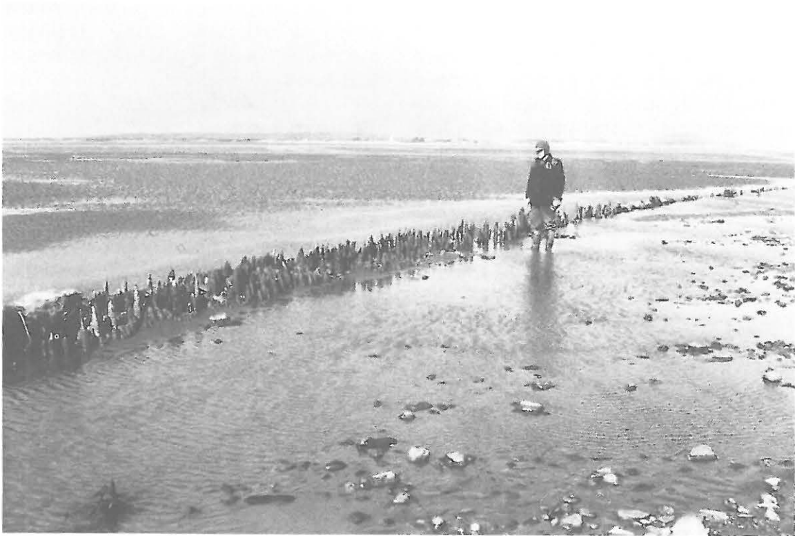
Figure 39. Part of the large, wooden walled fish weir (045), facing north east and on the south side of the Gutterway. This arm of the weir was at least 200 m long.
