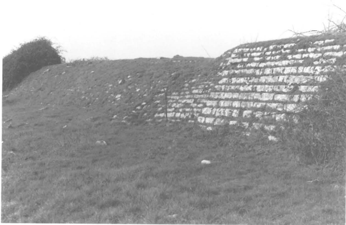
Figure 4: Seabank of 1590/91 with protective stone pitching.
