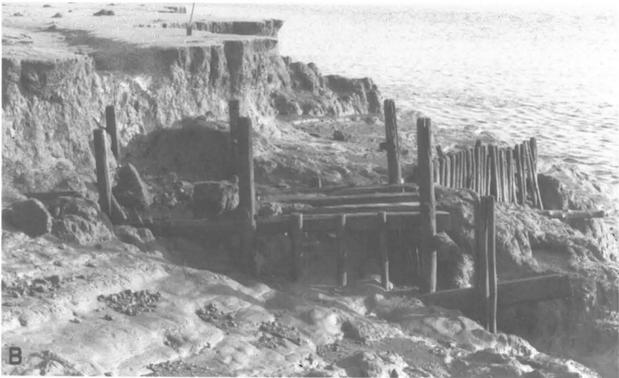
Figure 2: Views of the wooden jetties (spade for scale 0.94 m tall).
