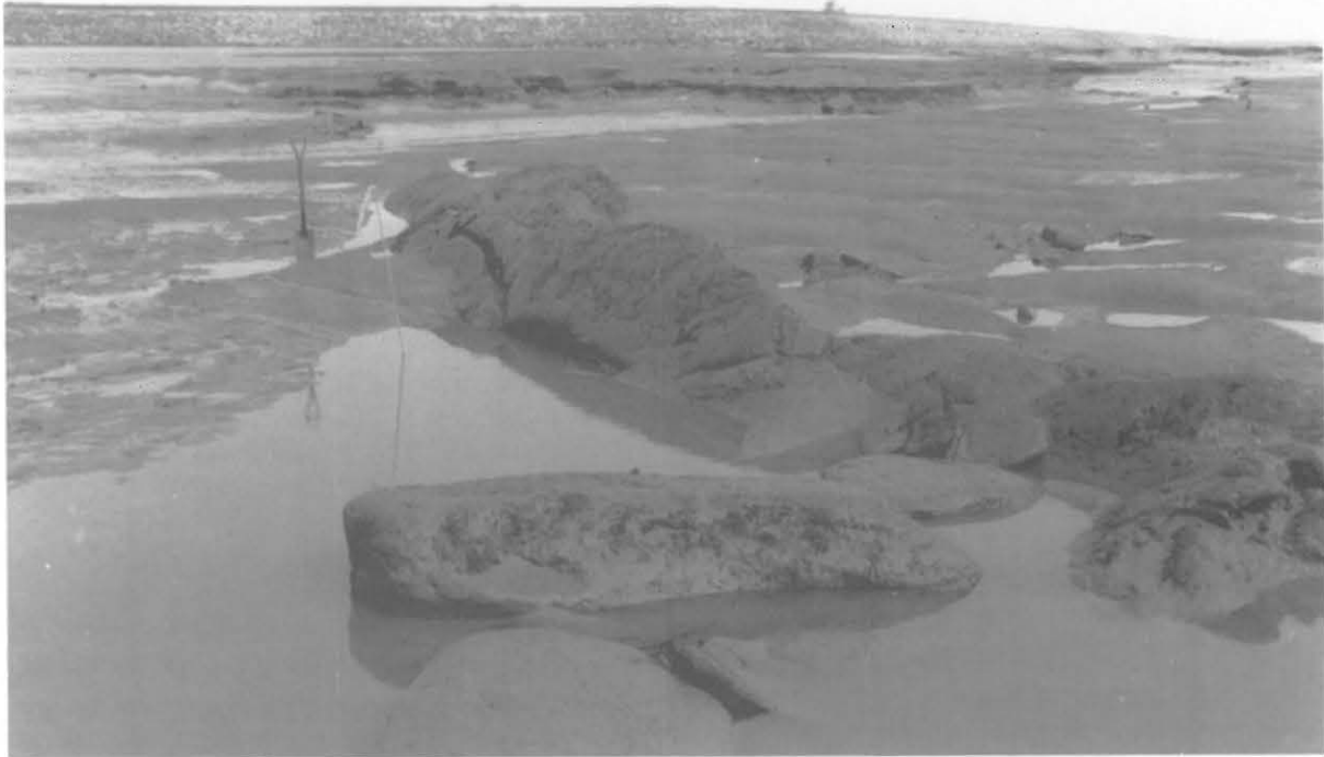
Figure 3: Toppling failure of silts and peats (arrows show dip direction), left bank of palaeochannel. Spade for scale 0.94 m long.
