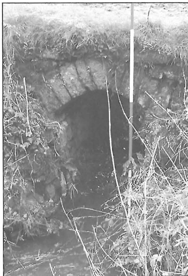
Figure 3: Stone vaulted tunnel under the line of the Bishop's deer park at ST 4705 4755.
