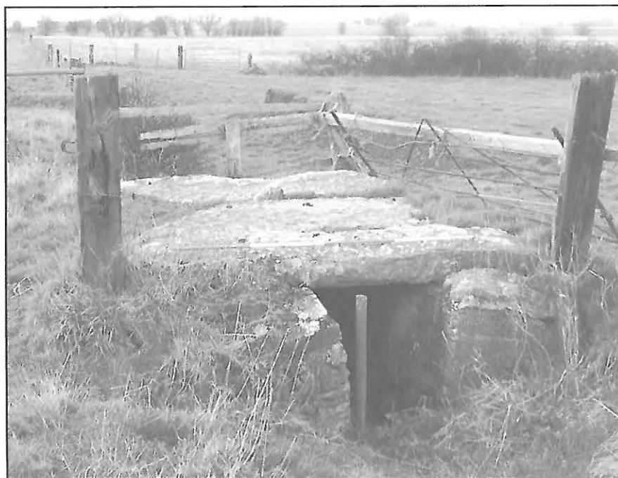
Figure 4: 'Clapper' style stone bridge over Gooseland North Rhyne at ST 4821 4736.
