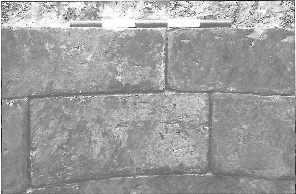
Figure 6: Detail of the ashlar masonry.
