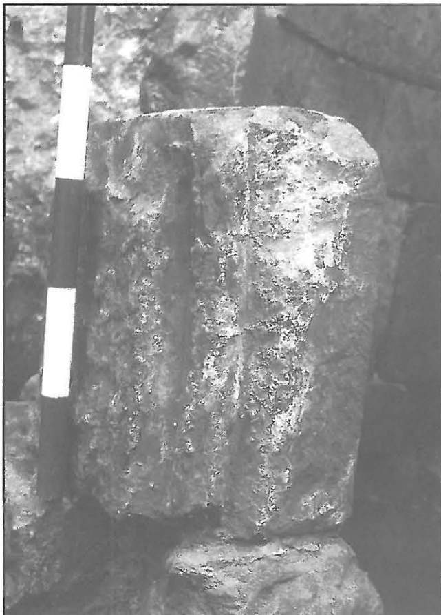
Figure 7: Voussoir in position.
