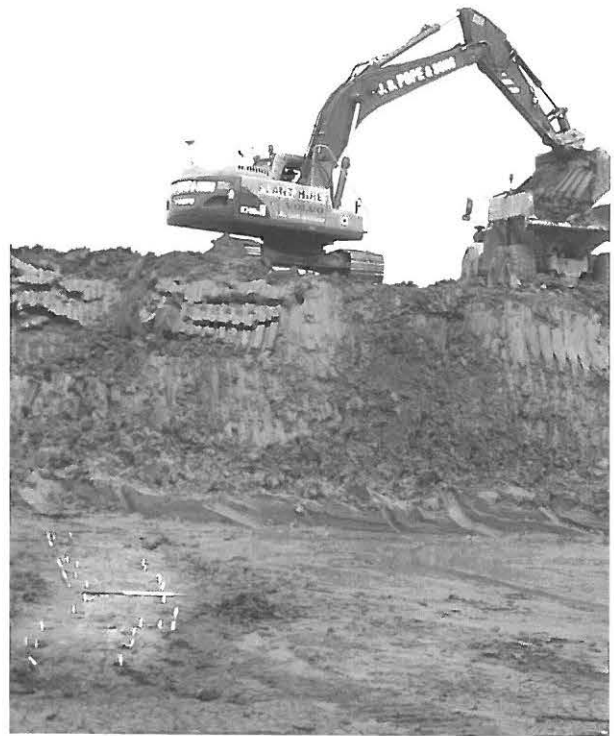
Figure 11. Structure 4, general view looking north.
