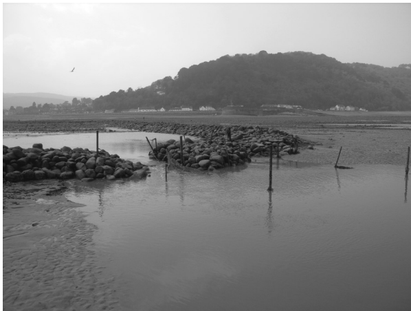
Figure 13 Metal scaffolding poles and modern netting by the 'gut' or outflow channel of a stone weir at Minehead Bay, Somerset.
