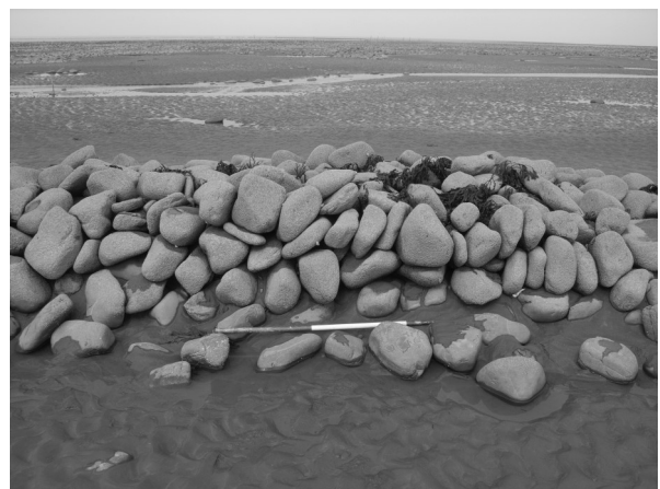
Figure 15 A well-built, coursed stone leader arm of a stone fish weir at Minehead Bay, Somerset.
