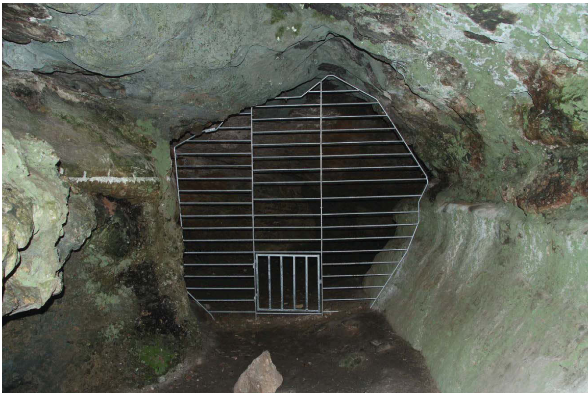
Figure 2.3.2. The grille after installation.
