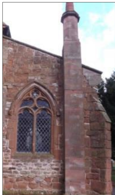
Fig 36: Chimney on south aisle
