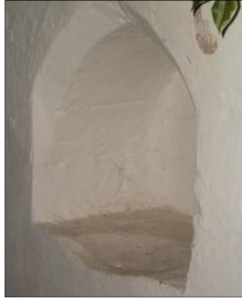
Fig 22: Broken piscina in the south aisle possibly the location of the 'Chapel of the Blessed Mary of Grandborough'. A formerly projecting basin has been faced off.
