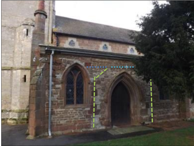
Fig 5: The south aisle, partly obscured by a yew tree; note the scarred stonework around the doorway where a former porch once stood (green dashed lines), the top of the scar itself removed by later roof repairs (blue dotted lines)
