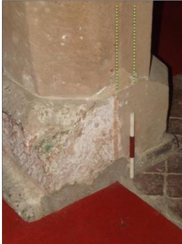
Fig 30: Altered arcade pier base: traces of (probably) medieval red paint and the scars of a removed vertical partition, possibly a tomb or chantry-railing at the west end of the south aisle; scale 30cm
