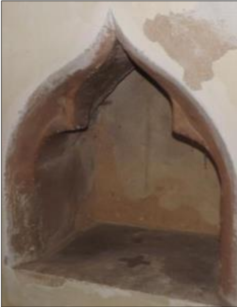
Fig 21: Principal piscina in the chancel. The drain is filled in
