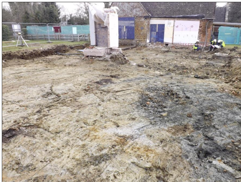
Fig 5: The site during mechanical stripping, looking south west, natural clays exposed. Existing cabling retained to the left of the brickwork. The existing foul sewer manhole is to the far right.
