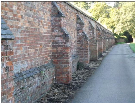
The heavily-buttressed north-west wall
