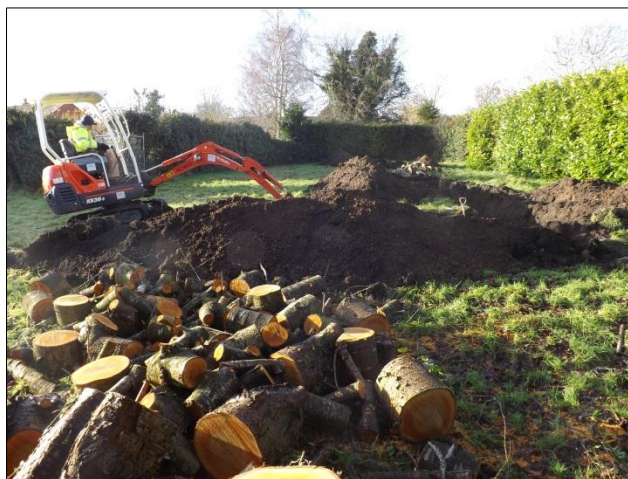
Fig 3: Excavation in progress, looking west .
