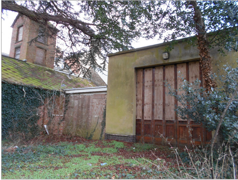
Fig 4: The rear of the buildings, looking south-west
