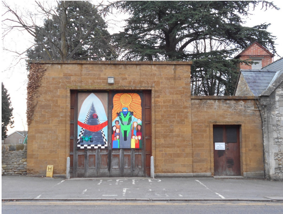
Fig 14: The later, flat-roofed extension adjoining
