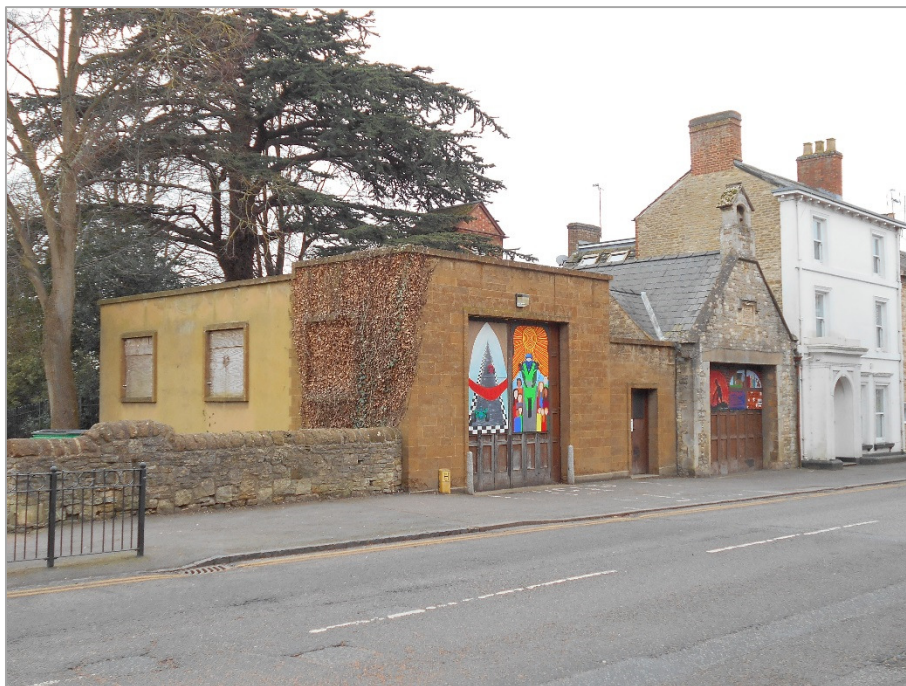
Fig 3: The old Fire Station buildings, looking south
