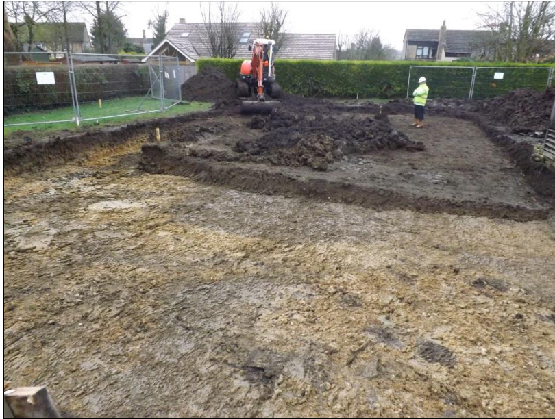
Fig 5: Mechanical site strip in operation
