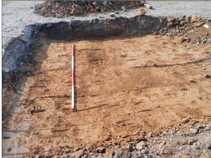
Fig 7: Trench 5, changed from a 10m x 1.6m trench to a 3m x 3m box to avoid live services. Looking north; Scale 2m
