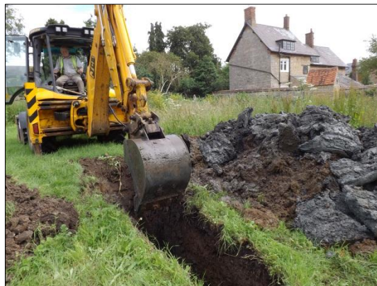
Fig 7: Geotechnical test-pitting; in the background is the Grade II-Listed 6 High Street.
