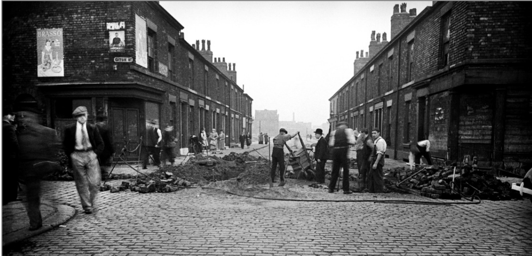
Fig 22: Junction of Caton Street and Duke Street, damage after bombing, prior to the Christmas raids of 1940 (Archives of the Greater Manchester Police)
