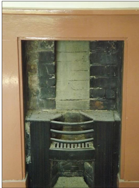
Fig 25: Probably an original fireplace and grate of 1811-17 in Bedroom 4
