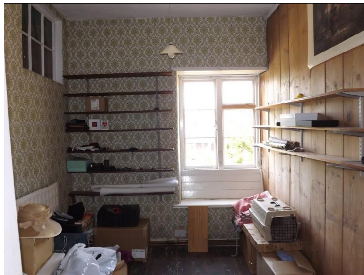
Fig 24: Board-partitioning (right) of the first-floor bedroom above the kitchen. The boarding bisects the only window. At top left the borrowed light into the store.
