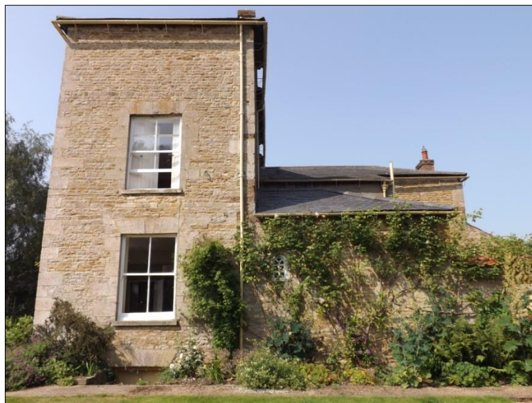
Fig 10: Geddington Grange Farmhouse; east face, its rear wing behind shrubs
