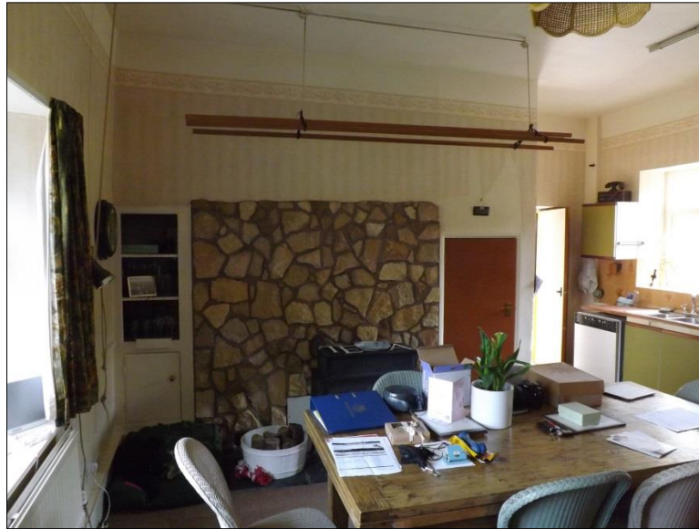
Fig 18: The kitchen – in-filled inglenook. To the left, the original (splayed) window location, to the right, the 20 th -century inserted window.
