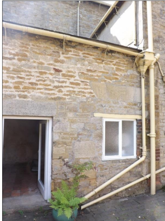
Fig 13: North-east wing: north wall.
