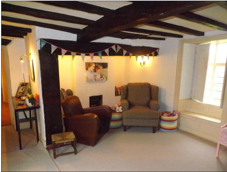
Fig 17: Sitting room G3 inglenook, note full shutters to right. A fire-light window has been blocked behind the armchair.
