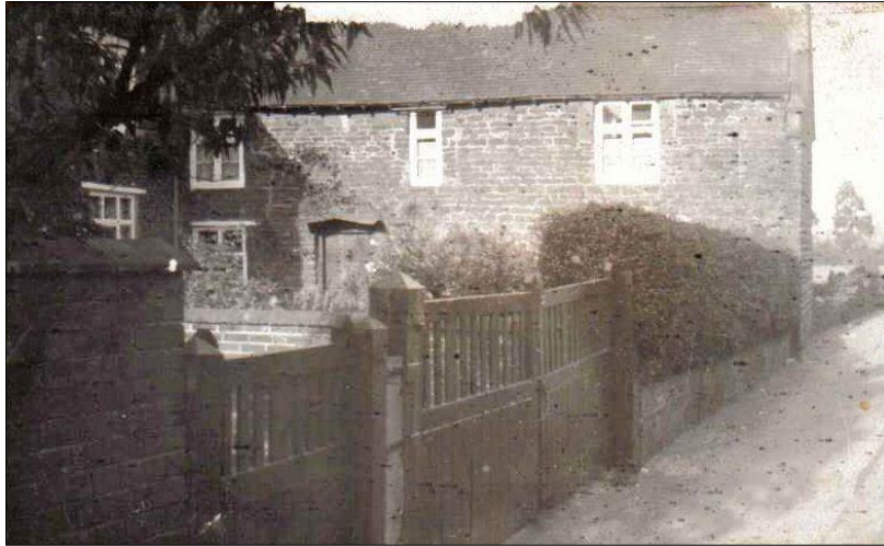
Fig 7: The clearest older view of the house, 1950s; note the old front door
