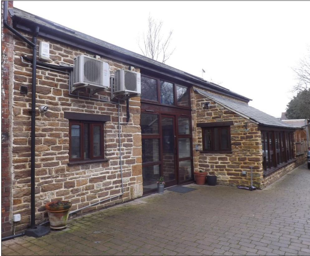
Fig 11: Detached barn, converted into a nursery and extended in the last decade.
