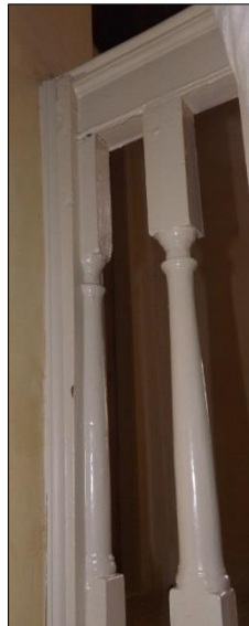
Fig 21: The handrail and stair balusters, possibly 18 th century.
