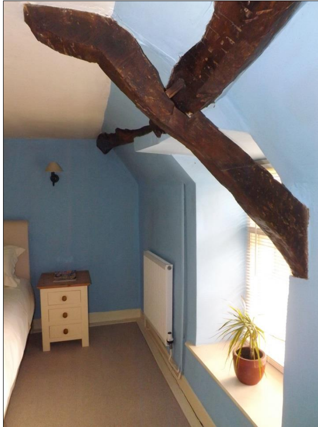
Fig 22: Bedroom F2, typical of the modernised finished interiors upstairs, but note the absence of a tie-beam. The wall-fast shoes of the truss ends have been strengthened in stone, visible on the outside.
