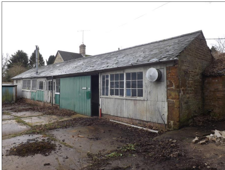
Fig 5: The adjacent former cart-shed, later garage office and workshop; scale 1m
