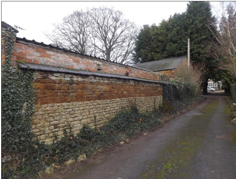
Fig 7: The farmyard eastern wall, distinctively of both limestone and ironstone, later raised in brick for the garage. The east end of the barn is glimpsed beyond. The row of overgrown Leylandii and two mature Sycamores behind had to be felled before the north side of the barn was photographed.
