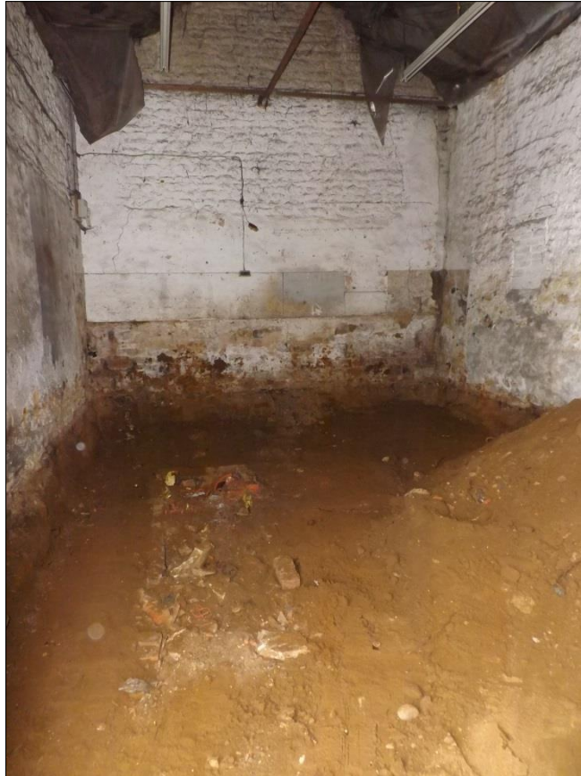
Fig 10: Western half of the barn; the vehicle inspection pit to left of centre, ground levels reduced.
