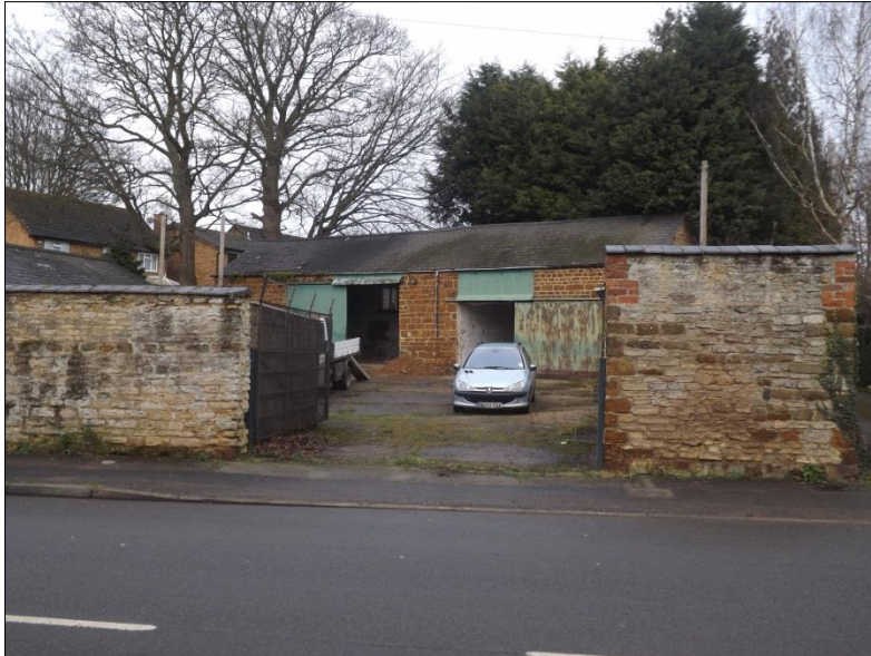
Fig 2: The barn and the courtyard in front, looking north, viewed across Church Street. Old photos show that the entrance was once flanked by substantial stone and brick gate-piers.
