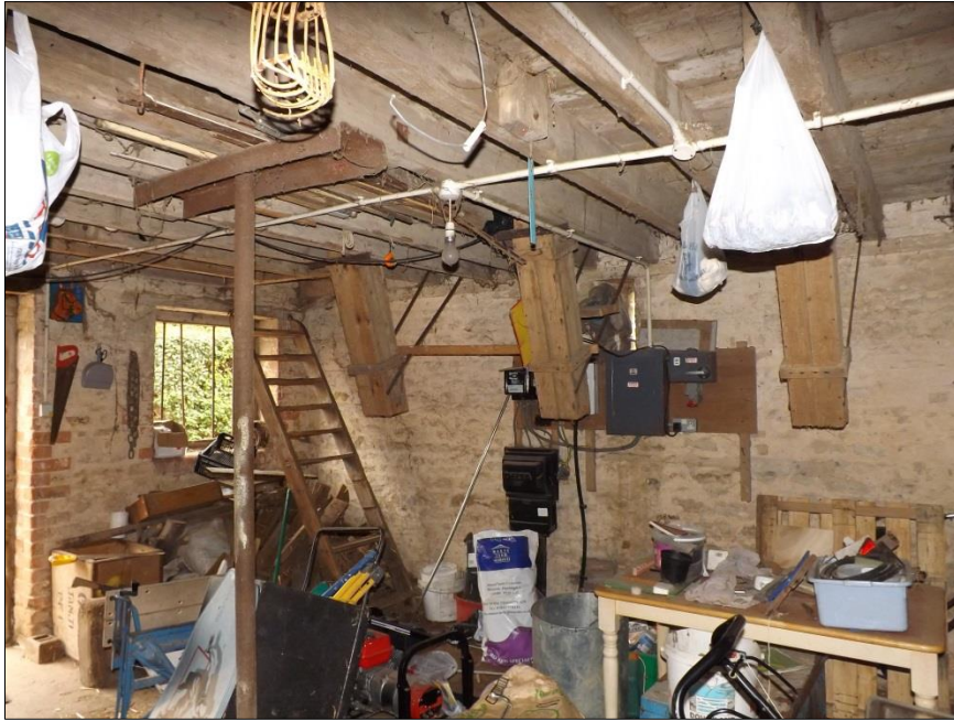
Fig 8: Ground floor interior, looking south-west towards the ladder access; note the three chutes, strapping and the iron ceiling strut
