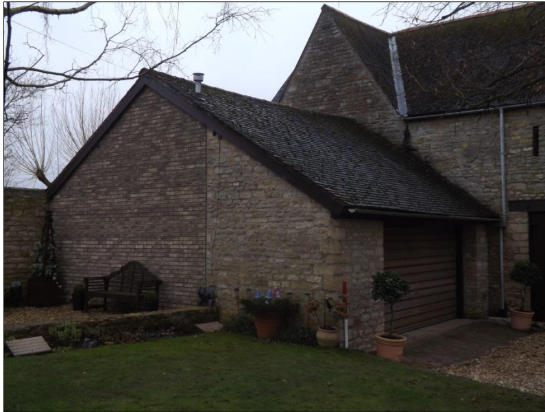
Fig 5: The added garage, partly occupying the footprint of an earlier agricultural building; scale 1m
