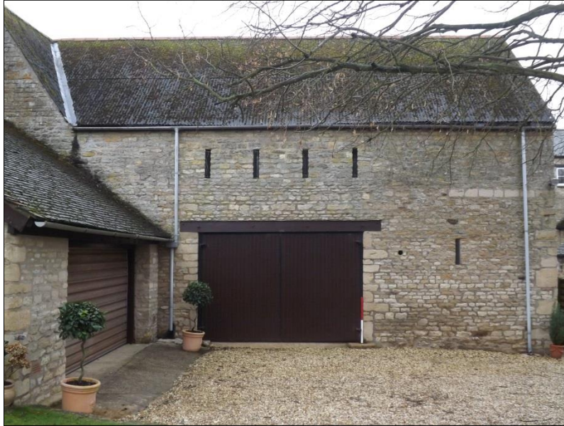
Fig 3: Mulberry barn from the north side. Note the inserted row of windows at first floor; scale 1m
