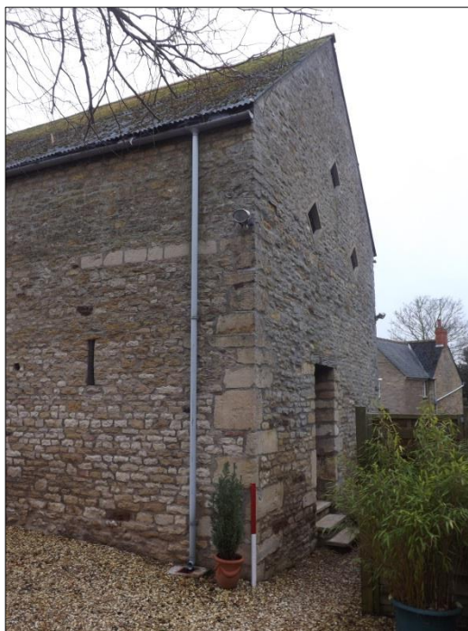
Fig 8: An ashlar course may denote a previous change. The west gable doorway is modern as are the gable windows; scale 1m
