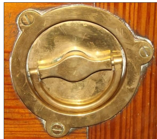
Fig 16: Folding/retracting brass handle to screen
