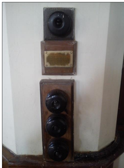
Fig 21: the 1930s or 40s Bakelite light-switches
