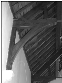
a: typical wall-post and hammer beam
