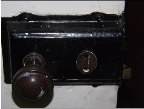
Fig 24: 1930s lock from servery to kitchen on door in Fig 21. Bakelite handle
