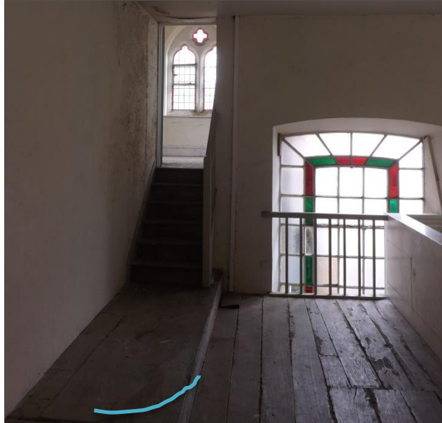
Fig 31: Gallery, looking north to the tower; note the curved timber edge in the step (marked)
