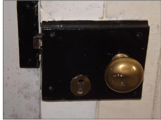
Fig 25: 1906 lock from servery to schoolroom on door in Fig 22. Brass handle
