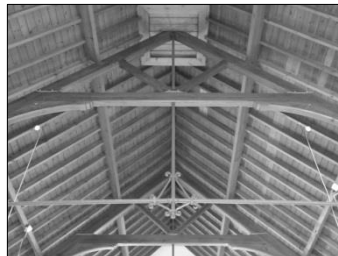
b: a typical truss, note the redundant base for a bell-cupola at top
