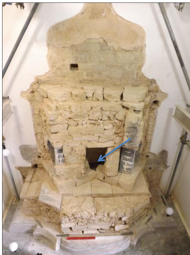
Fig 6: The monument core viewed from the dismantling gantry above; scale 1m. The apex of a low, flat arch hidden behind the monument is arrowed. The eastern spring of that same arch (on the far right here) can be seen in detail in the Figure below.
