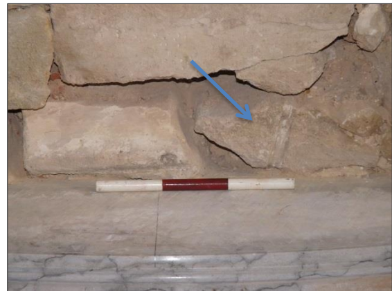
Fig 10: a better-preserved 14 th -15 th century cavetto mullion fragment still built into Stage 1 of the monument core (arrowed); scale 300mm
