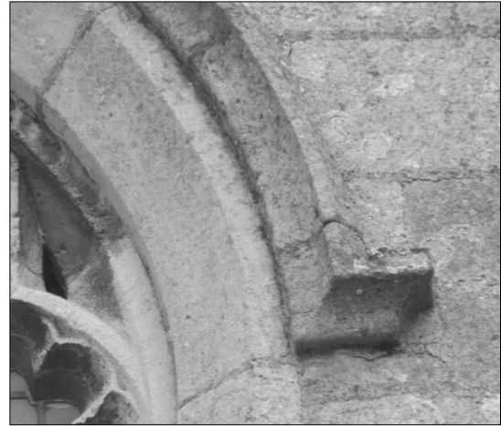
Fig 8a and 8b: Hood mould with label stop, and equivalent piece on St Edmund's tower; scale 300mm.
