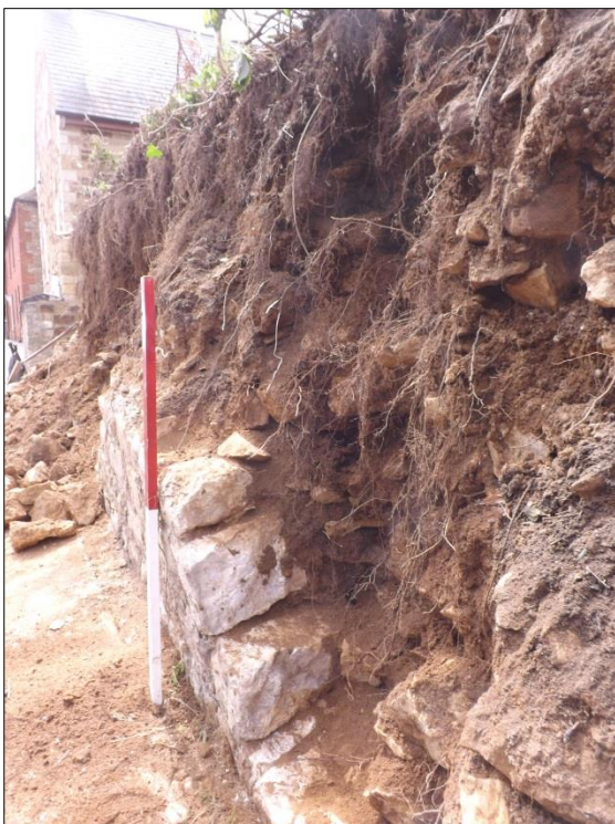
Fig 8: The section at 5m from the corner; note the collapse and thrust of loose soils which destabilised the skin; scale 1m.
