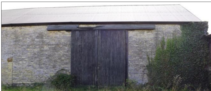
Fig 20: Barn B west annexe
