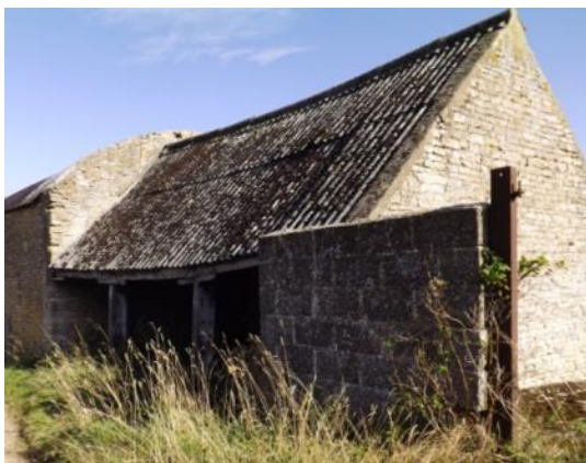
Fig 14: Barn A south annexe, exterior
