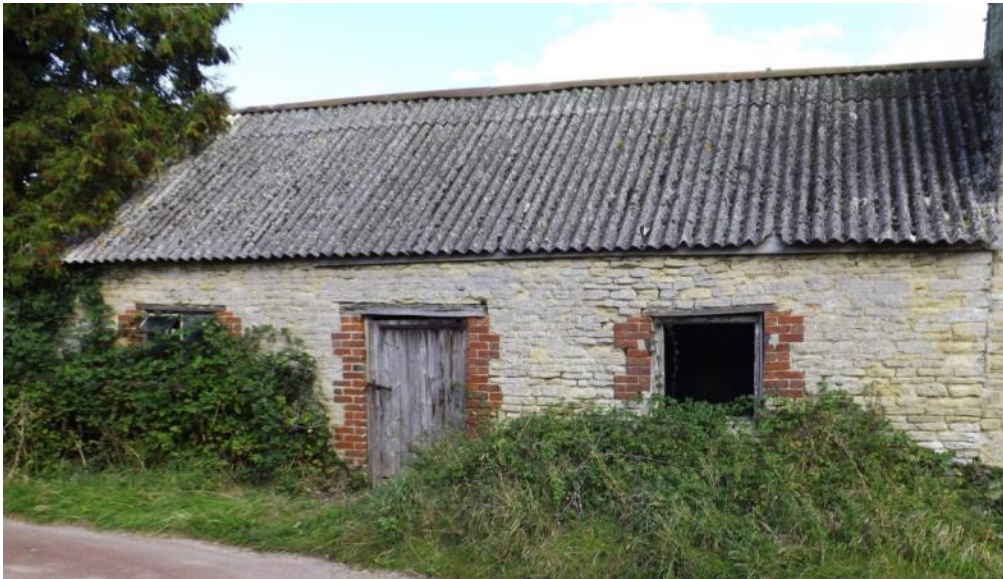
Fig 12: Barn A, north annexe, front (west) face; Barn A to right
