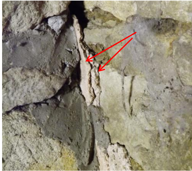
Fig 10: Former north-wall plastering layers, sandwiched at the north-west corner by the construction of the west wall
