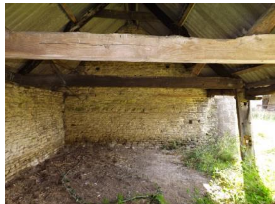
Fig 15: Barn A south annexe, interior
