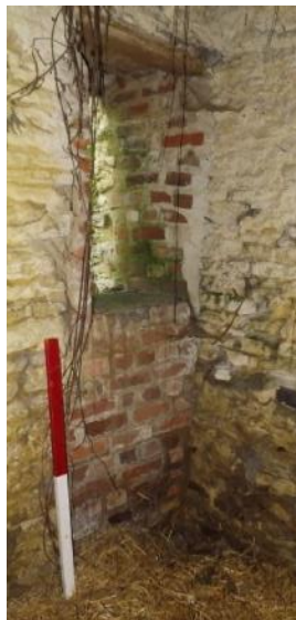
Fig 11: Threshing belt opening in north gable wall; scale 1m
