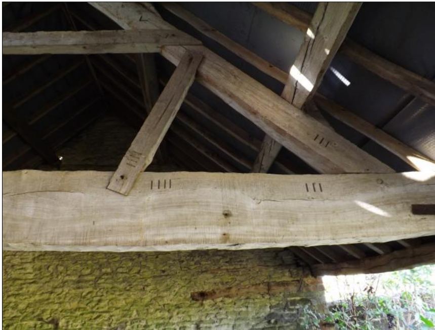
Fig 25: Roof truss in Barn D, showing carpenters' marks
