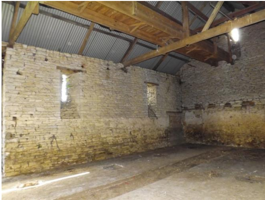
Fig 17: Barn B interior, east half. Note original ventilator windows, the high walkway and the silo/bin slots in floor
