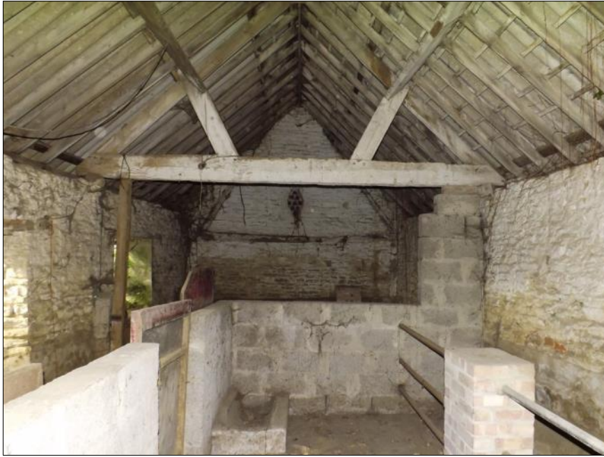
Fig 13: Barn A north annexe, interior, looking north
