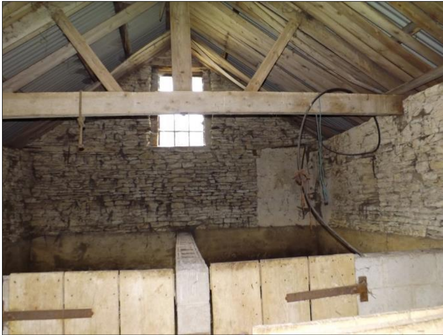
Fig 18: Barn B, east annexe; interior
