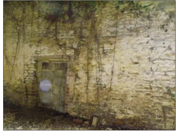
Fig 8: Blocked doorway north of cart doorway
