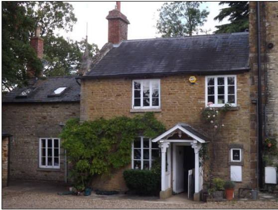
Fig 6: Kitchen range and service range set back to left (front, south, elevation)
