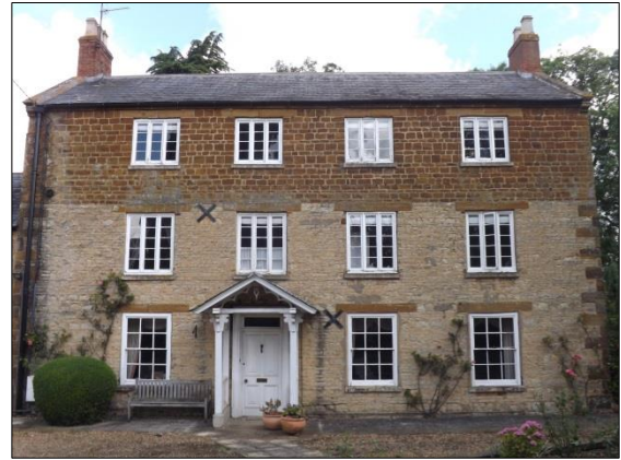
Fig 7: Main house, front, south, elevation; note the added second floor
