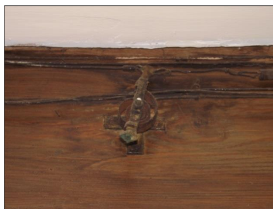
Fig 10: A bell-stump on the bell-board
