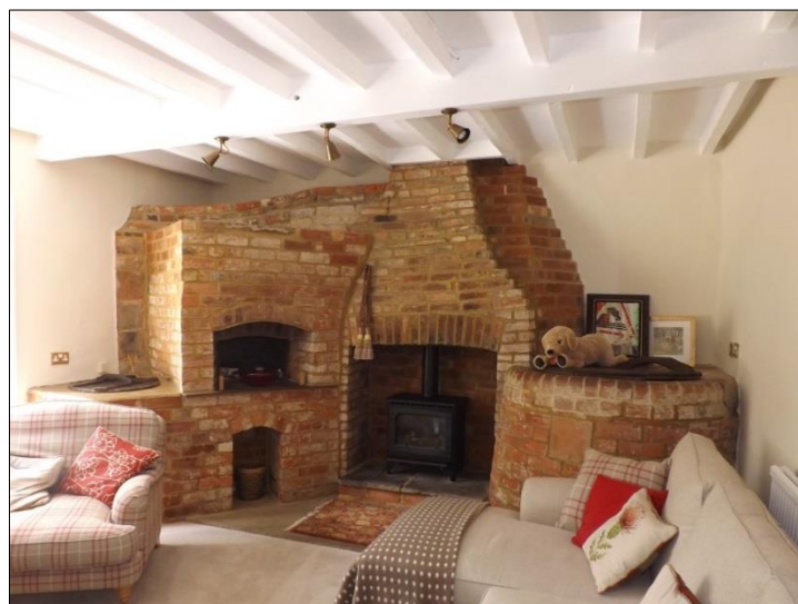
Fig 14: The beautifully-conserved service range with its end fireplace and added oven (L) and coppers (L & R)
