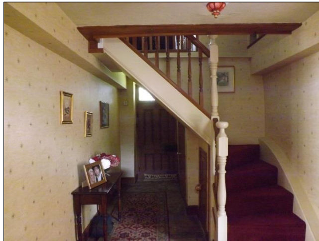
Fig 13: The awkward centre hallway, its route blocked by a stair and flanked by modern RSJ-topped partitions
